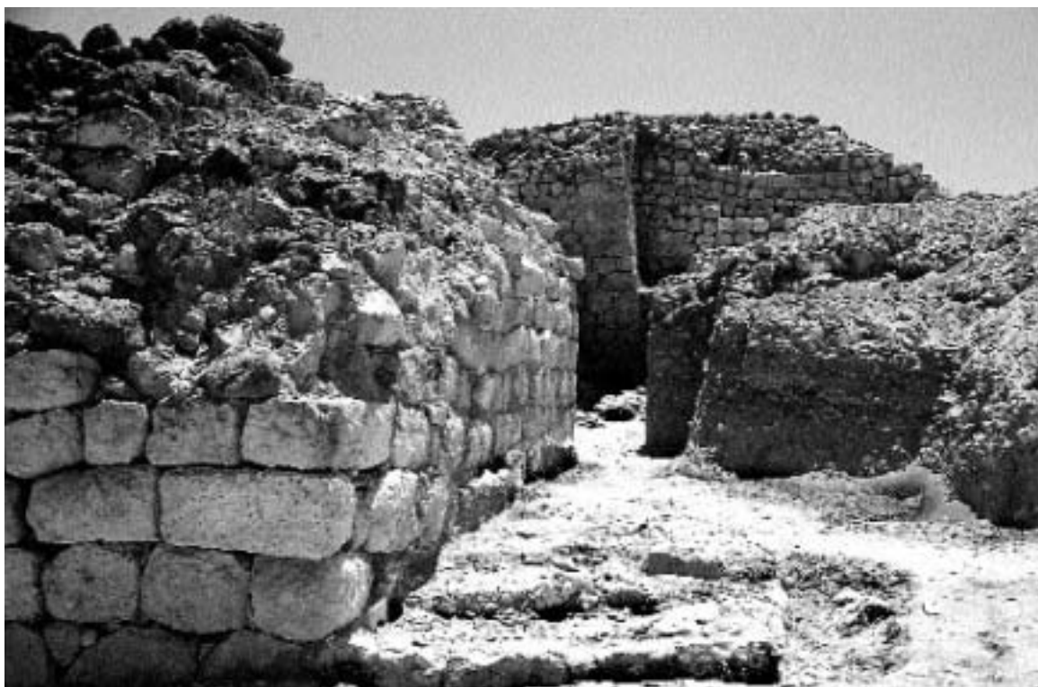
Fig. 6 - The stone platform connected with the turret M9.
