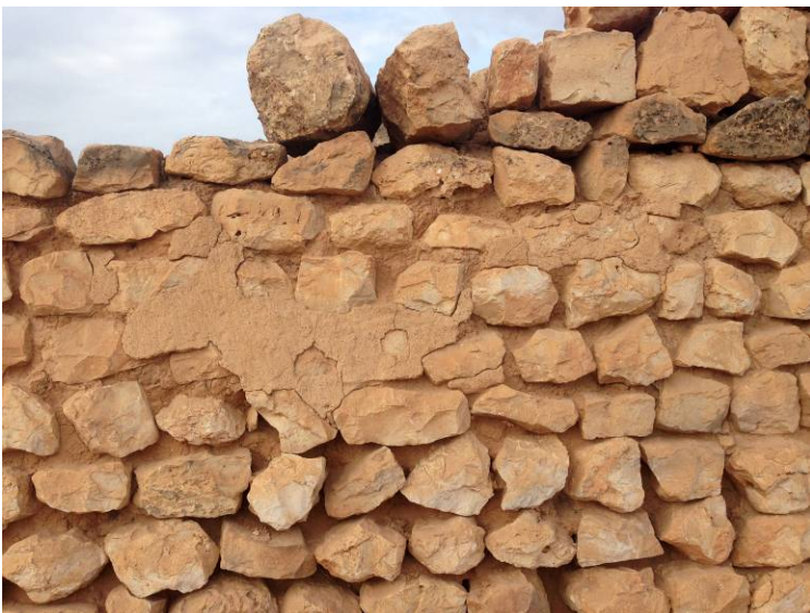
BF5 (north view): outer surface of M93 covered with plaster.
