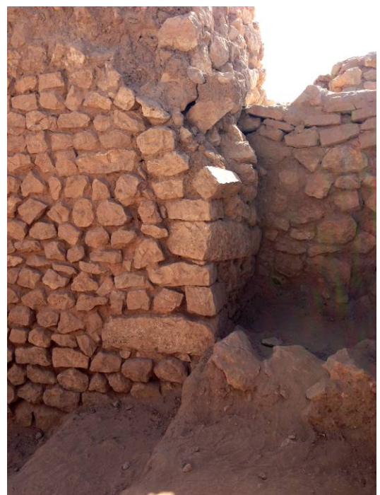
BF5 (south-west view): outer corner of MB2 with long cornerstones crossed.
