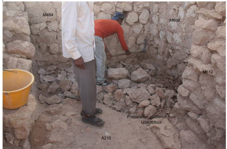
Removal of US636 floor with the preparation for the plaster.
