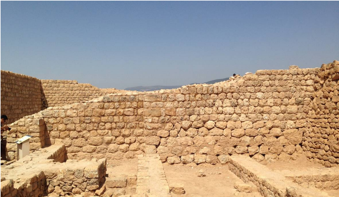
From East side
