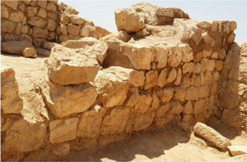
M529, north front wall after the restoration
