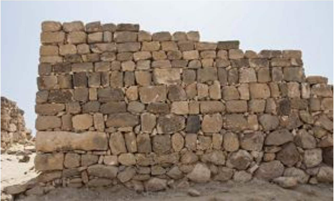
North side after restoration
