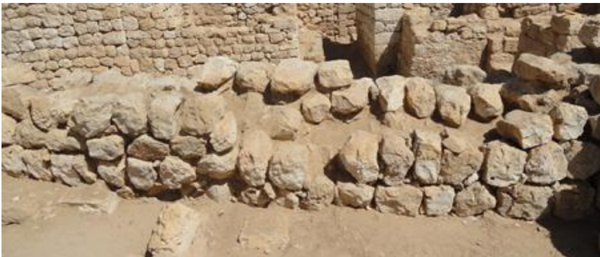
M485, north front wall, before the restoration.
