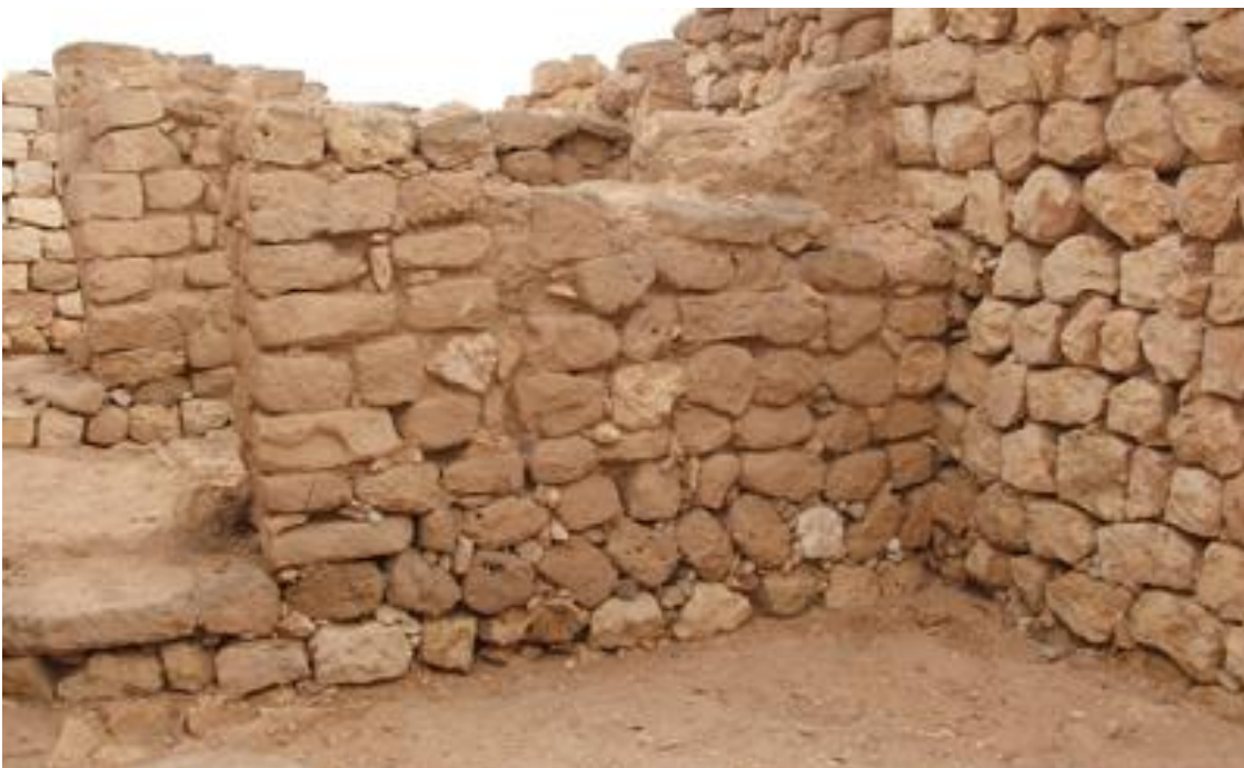
M77, north front wall, before the restoration.
