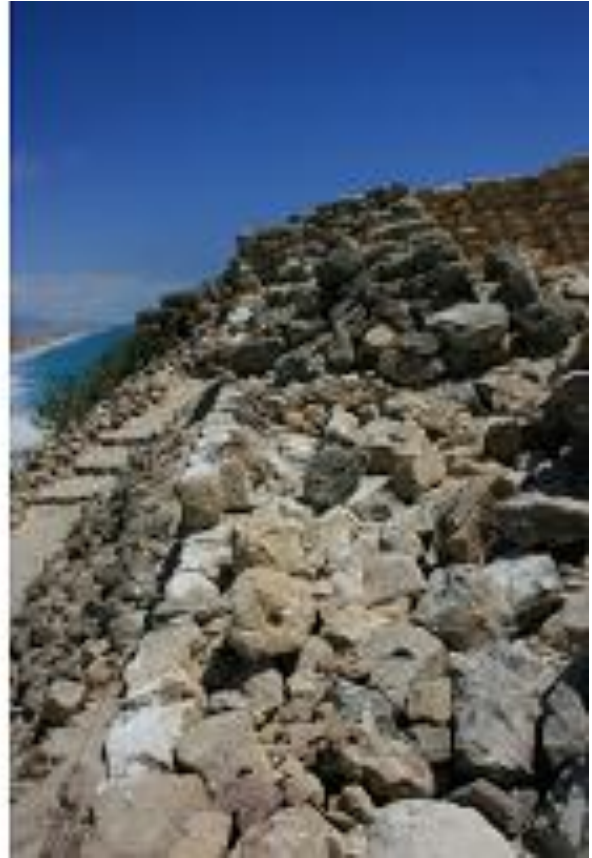
Construction of regular rows
