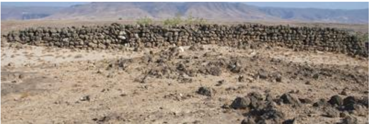
East wall in good condition
