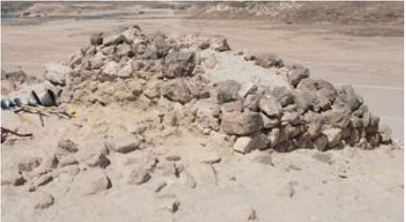
South side before restoration
