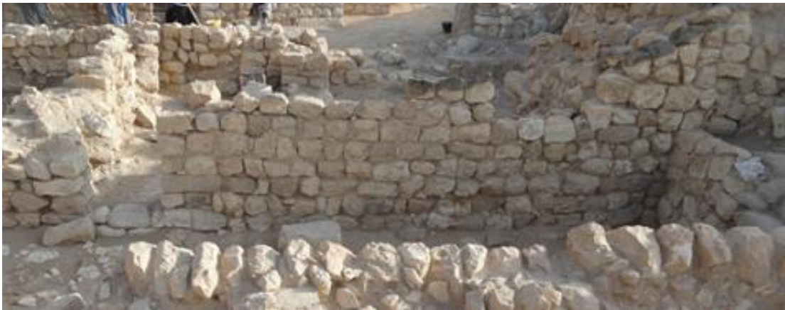
M581, south front wall, before the restoration.
