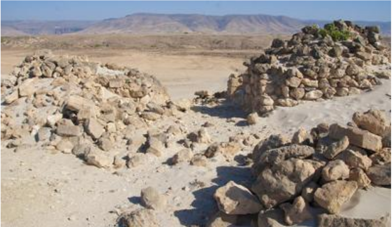
Principal door south side before restoration
