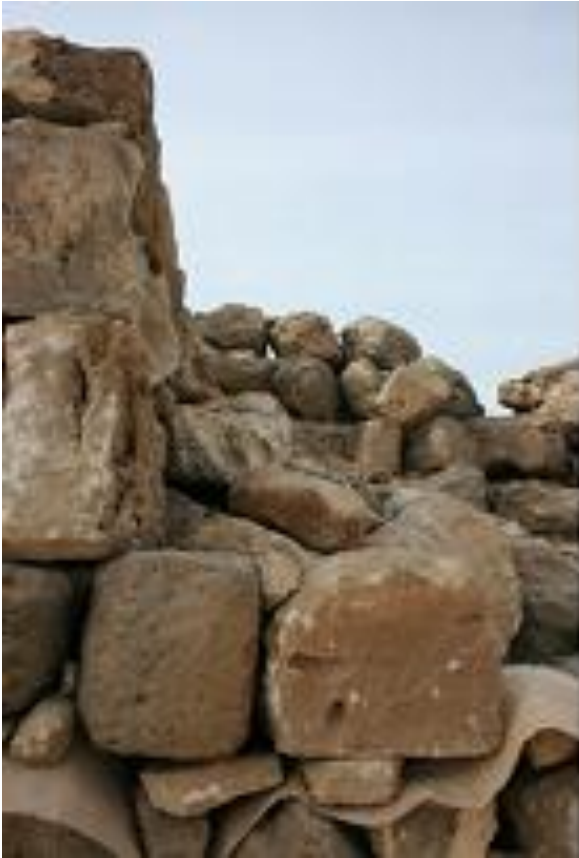
North face, connection with west tower
