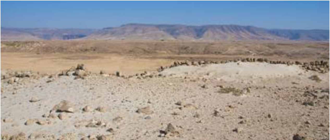
East wall in bad condition
