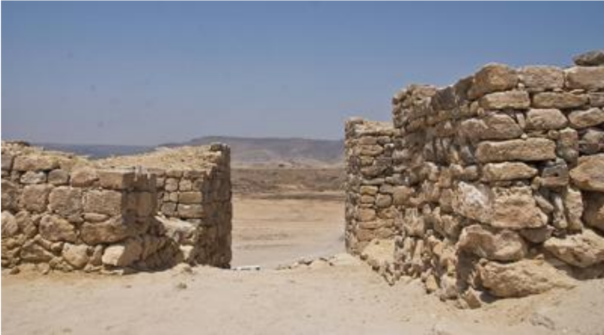
Principal door south side after restoration
