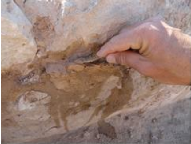
Laying of new plaster
