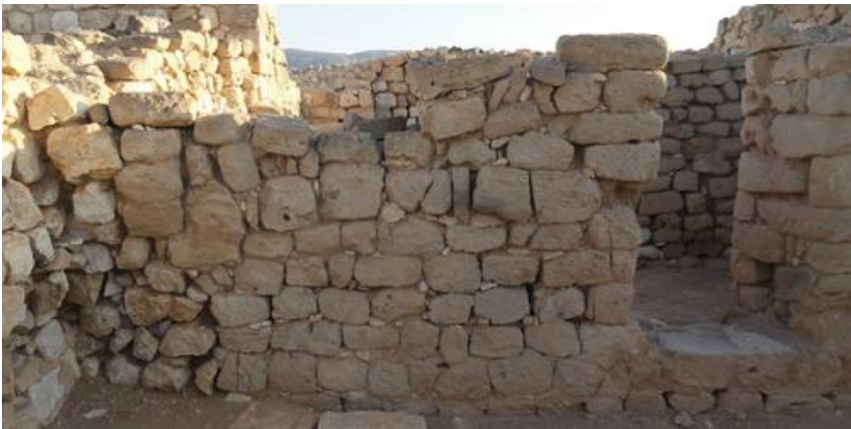
M70, south front wall, before the restoration.
