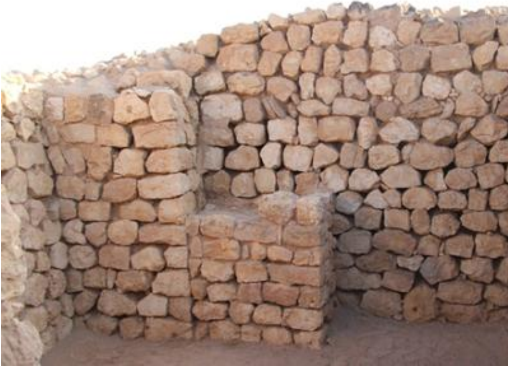
M69, south front wall, after the restoration.
