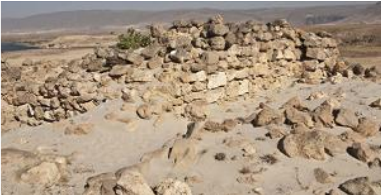
View south-west side before restoration
