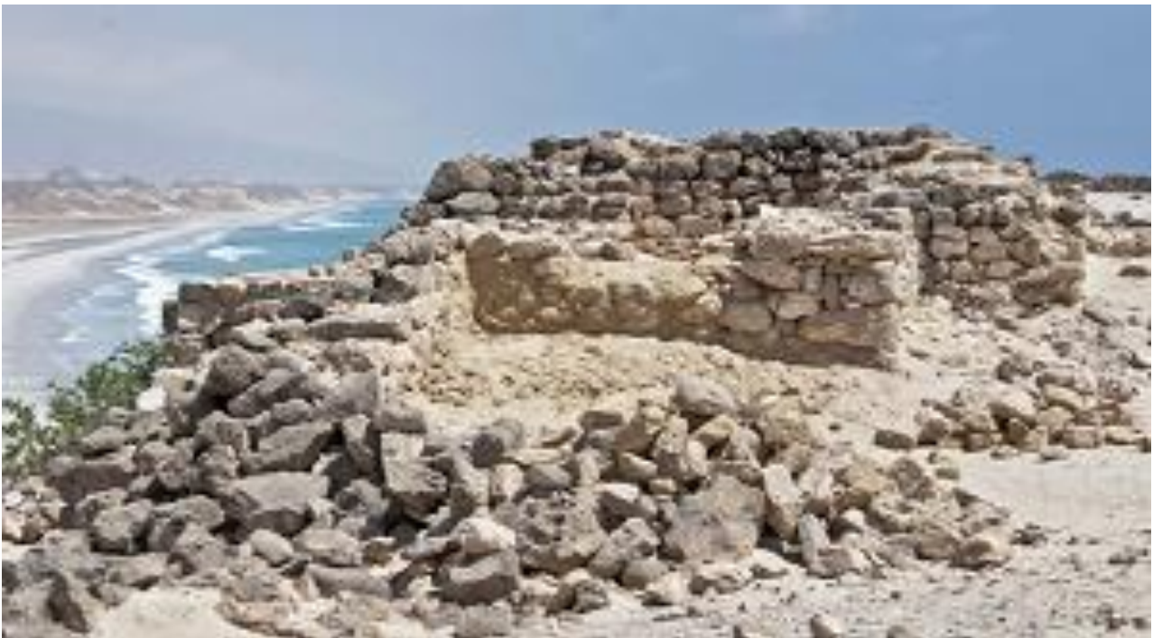
East side before restoration
