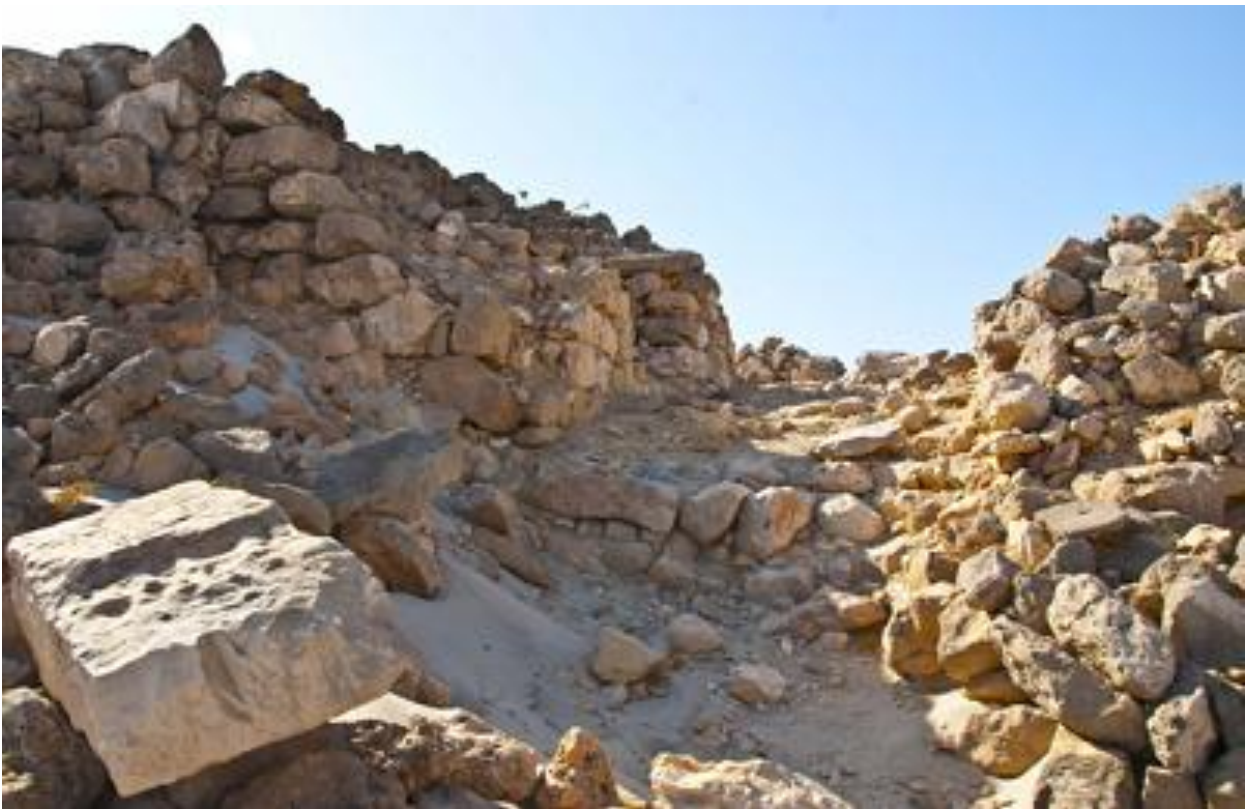
Principal door north side
