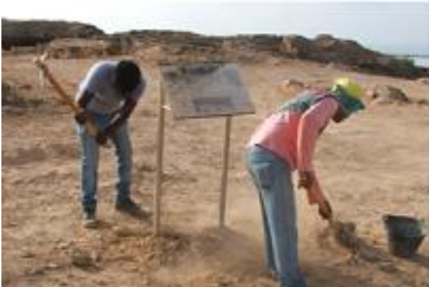
Removing the existing panel
