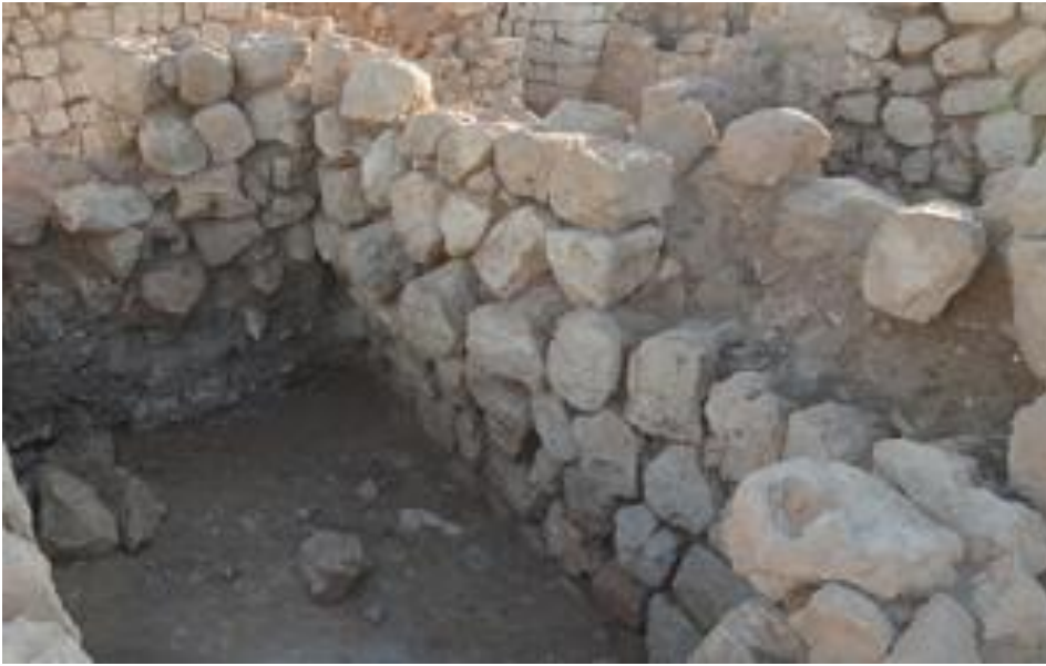
M494, west front wall, before the restoration.
