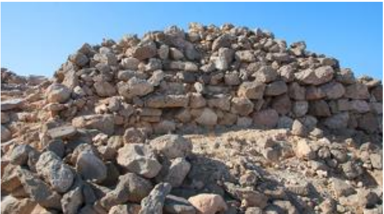
North side before restoration
