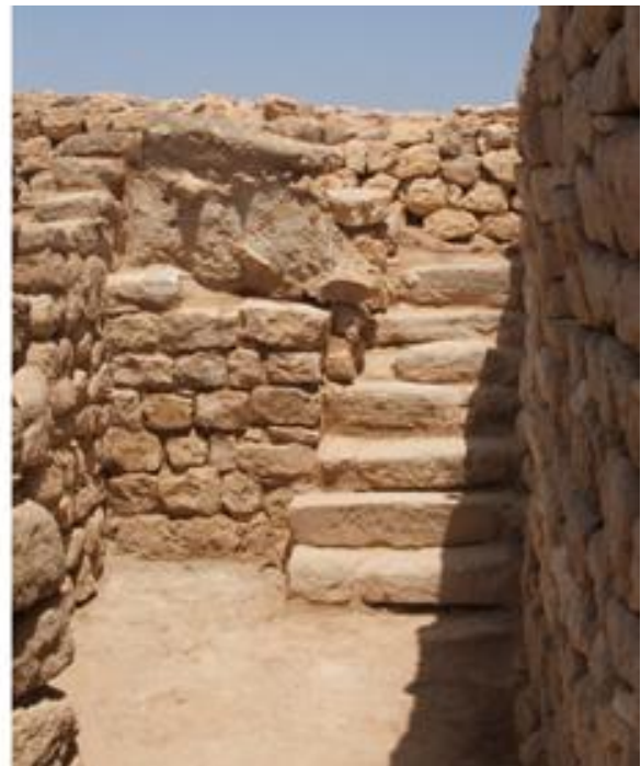
M63, south front wall, after the restoration
