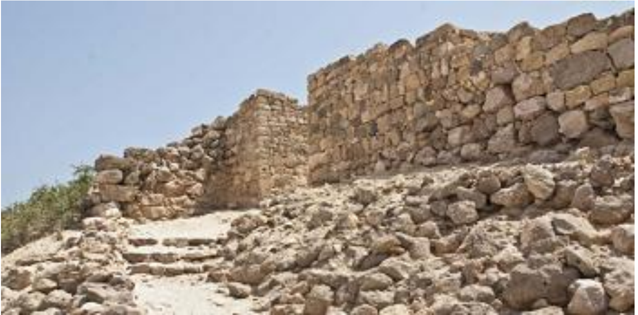
View on the up street after restoration
