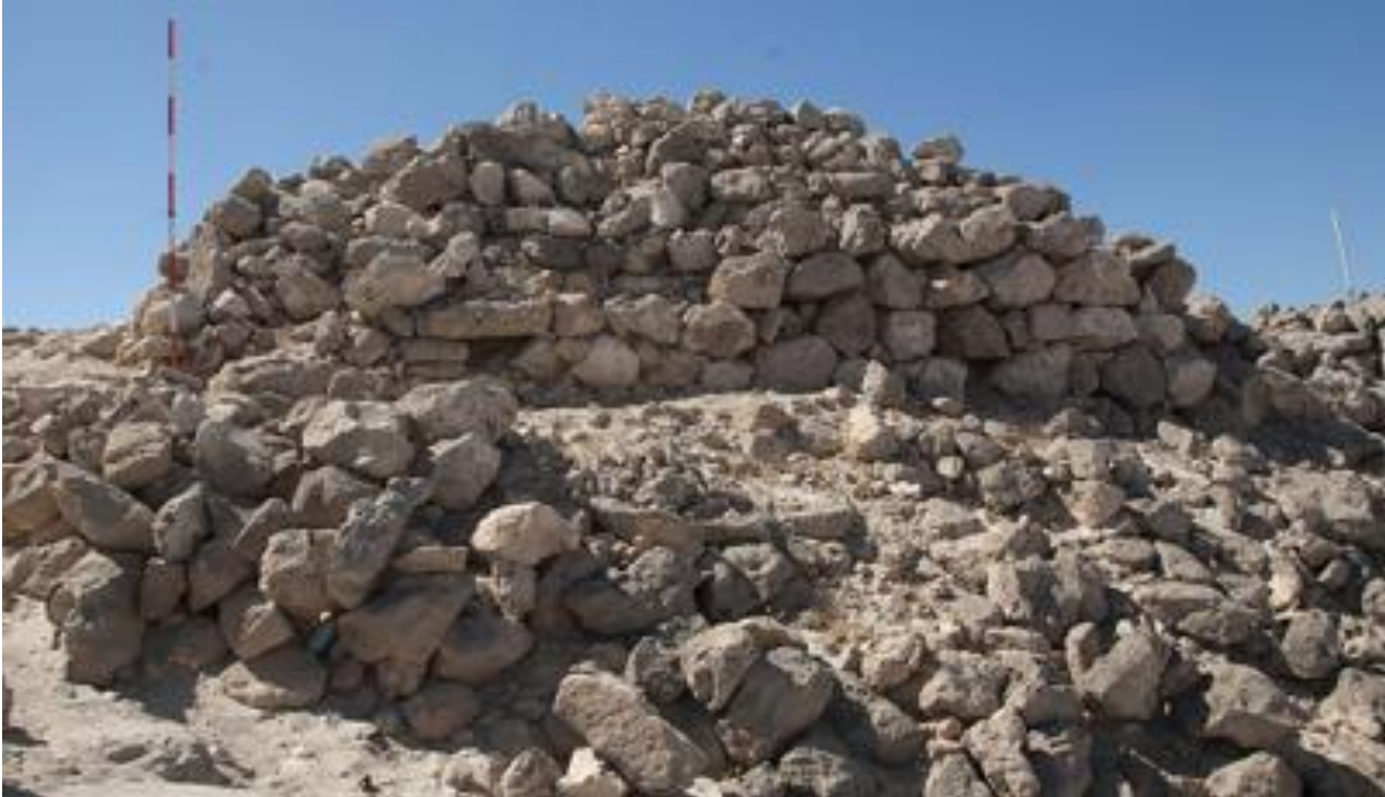
West tower north side
