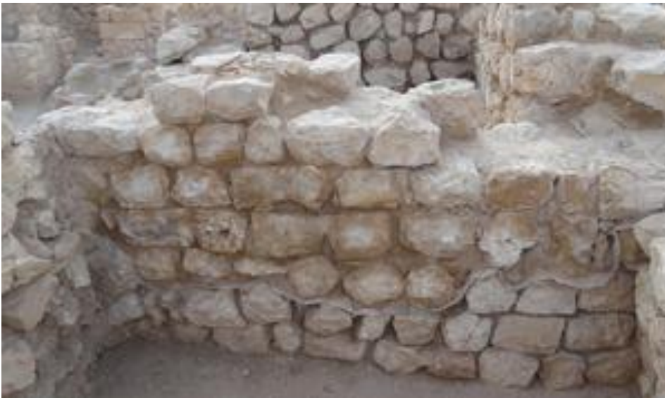
M494, west front wall, after the restoration.
