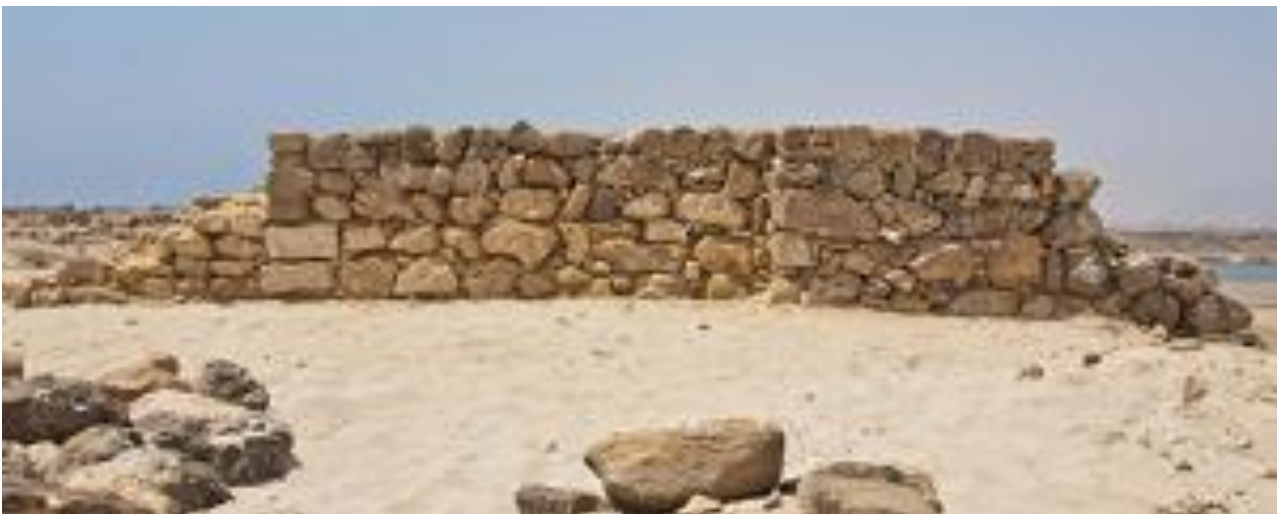
View west side after restoration
