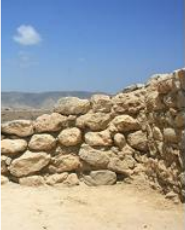
Connection with tower
