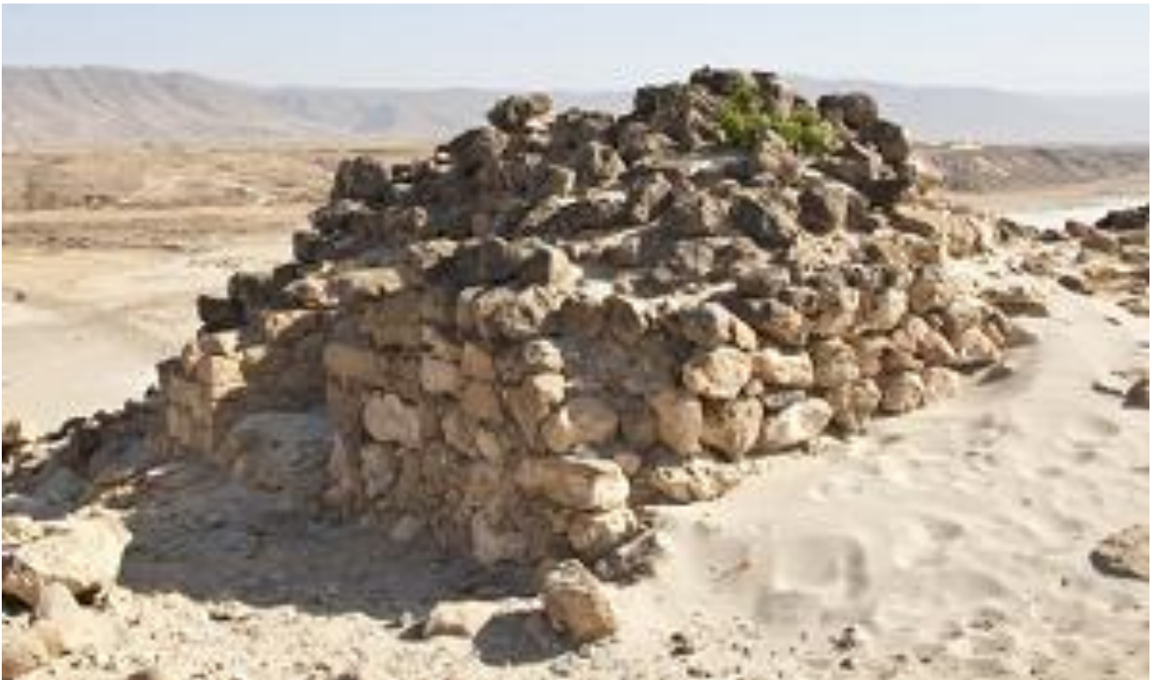
View east-south side before restoration
