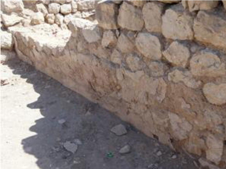
M494 (BA13), west wall, façade. before the restoration
