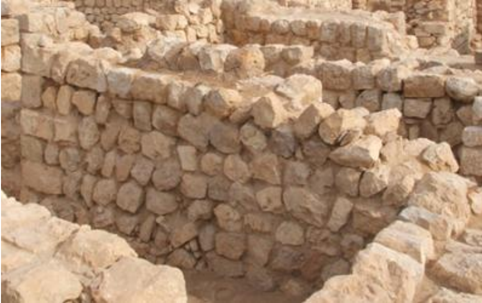
M562, north front wall, after the restoration.
