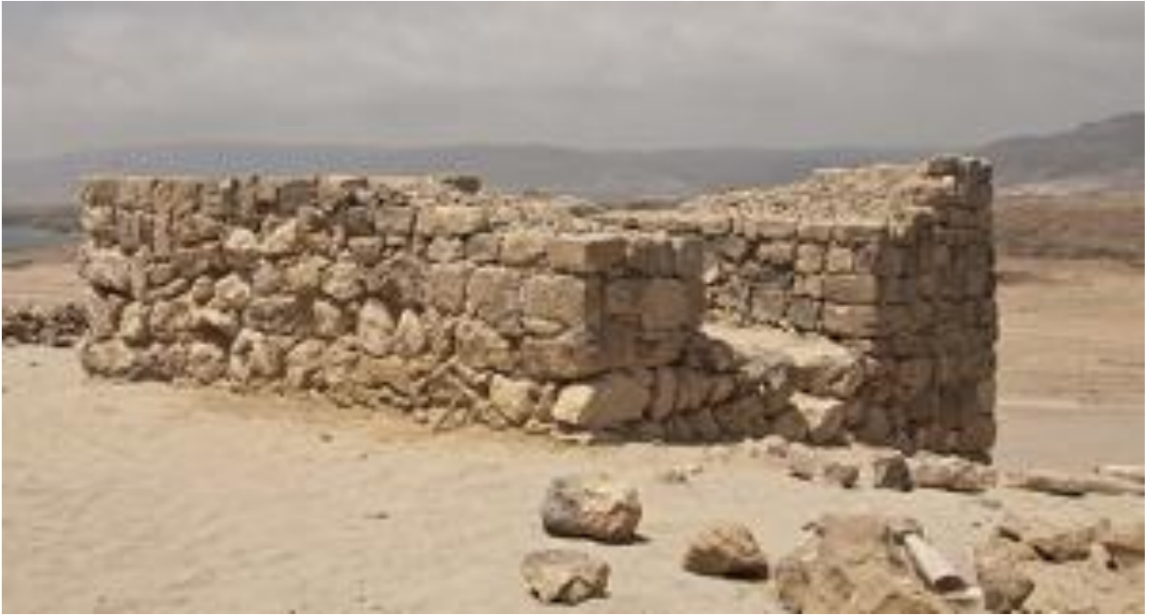
South side after restoration
