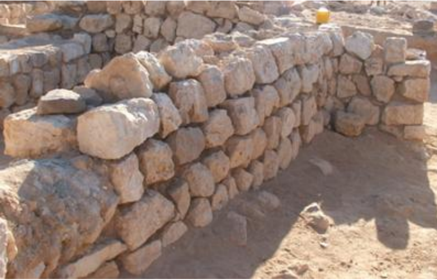
M569, north front wall, before the restoration.
