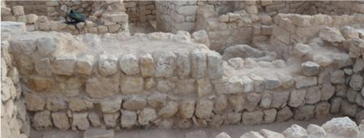
M485, north front wall, after the restoration.
