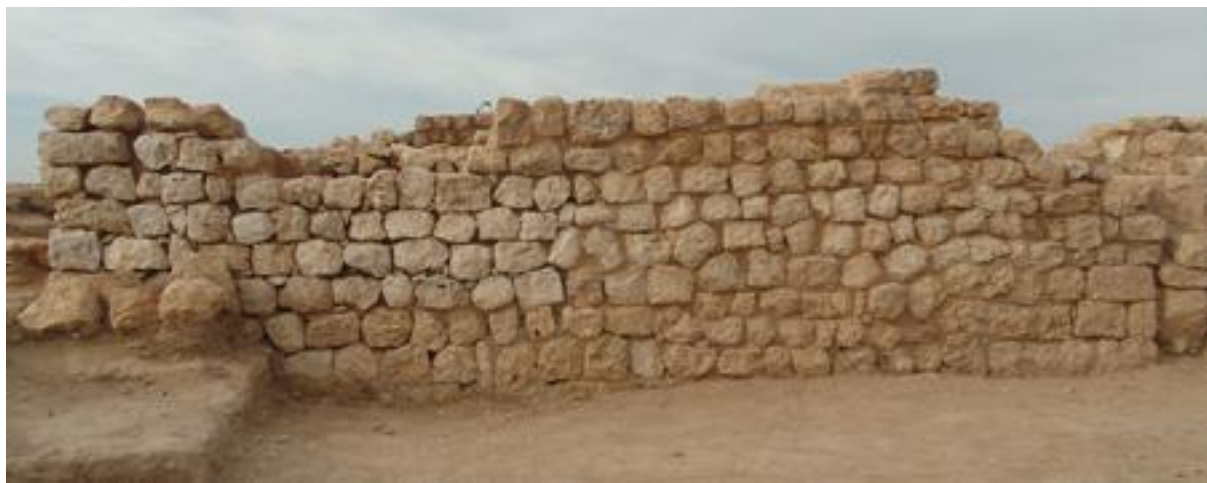
M485, south front wall, after the restoration.
