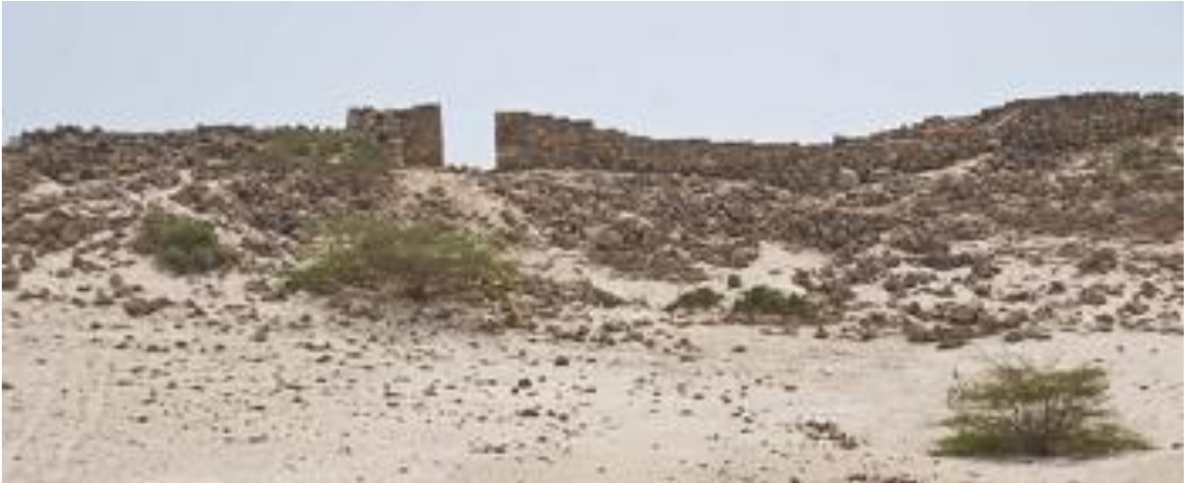
View on the down street after restoration
