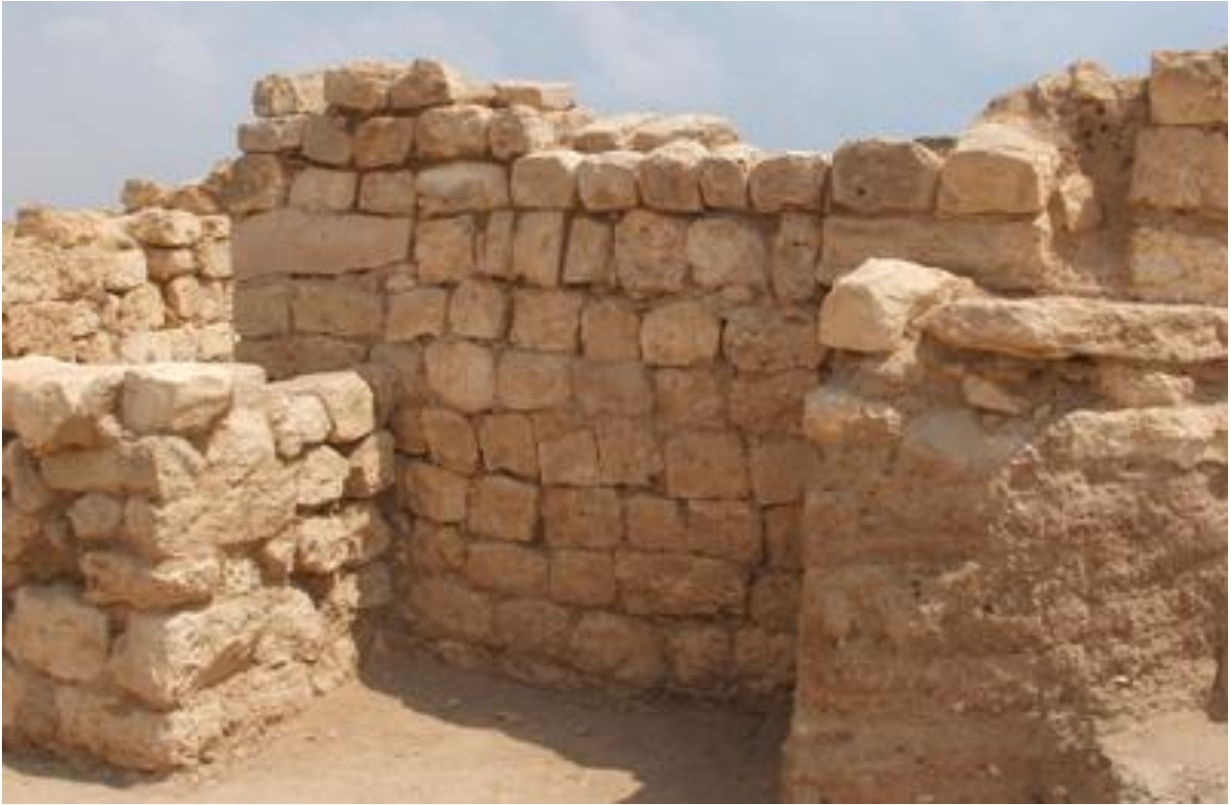
M521, west front wall, after the restoration
