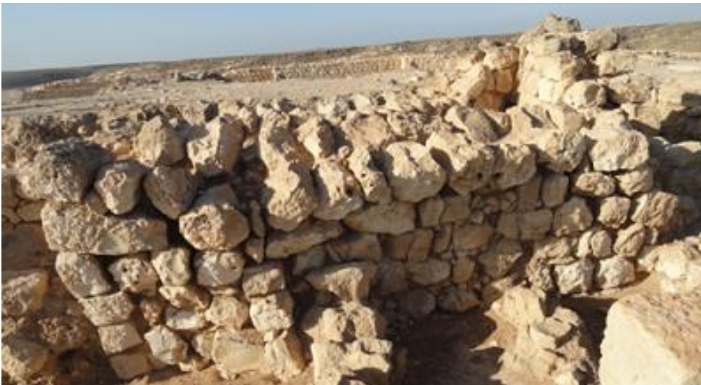
M567, south front wall, before the restoration.
