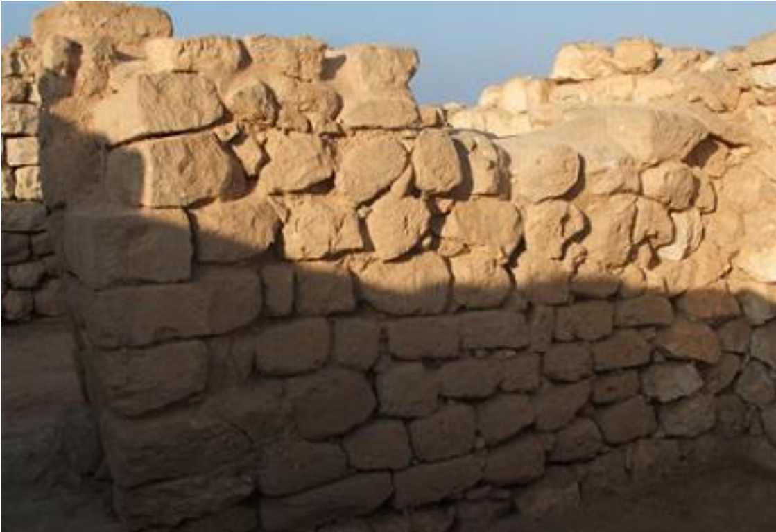
70, south front wall, after the restoration
