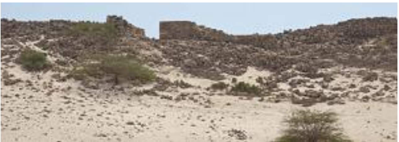
View on the down street after restoration
