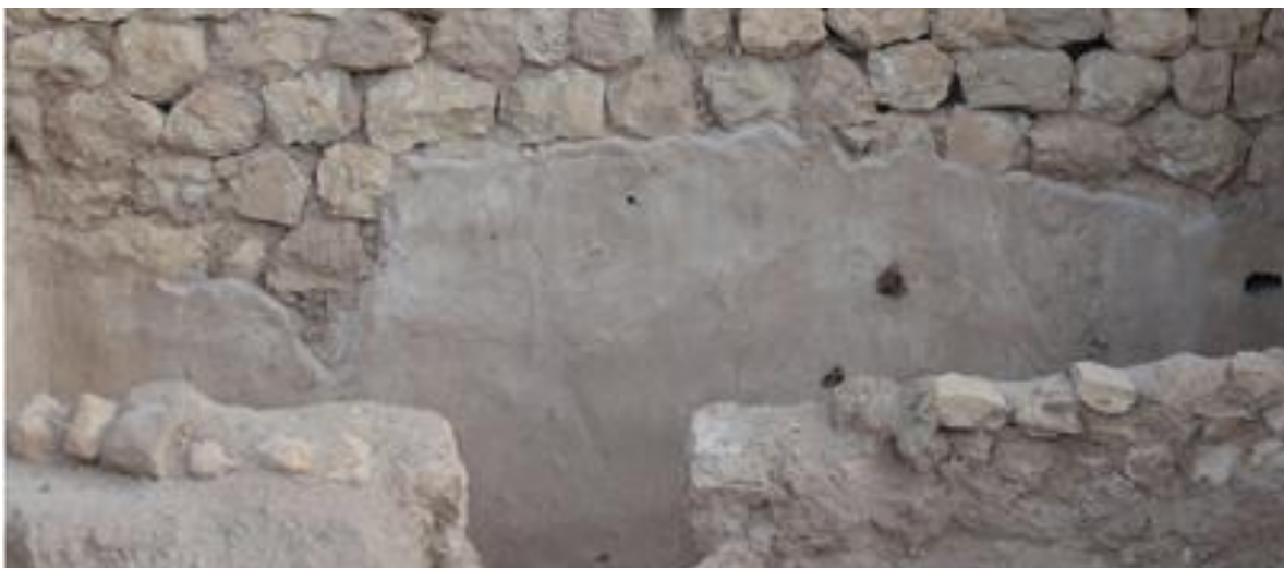
M17 (A121), south wall, façade. after the restoration
