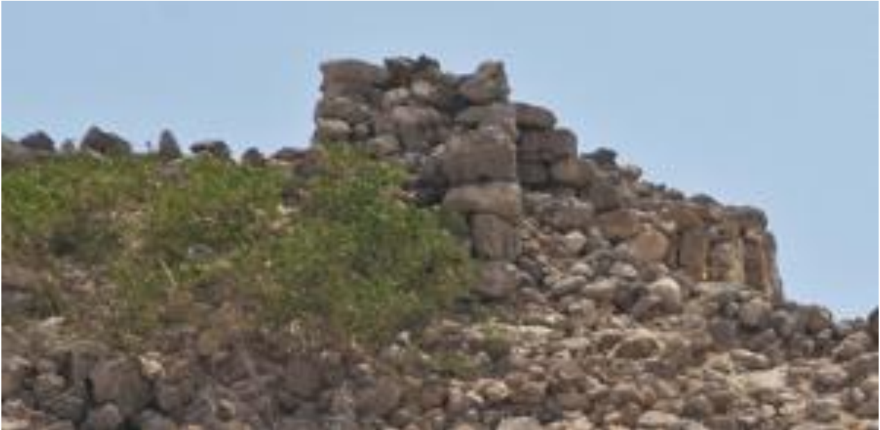
View north side before restoration
