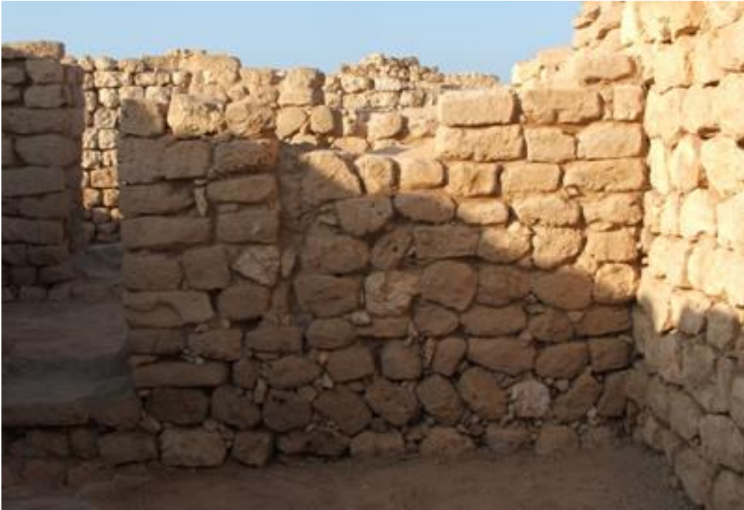
M77, north front wall, after the restoration.
