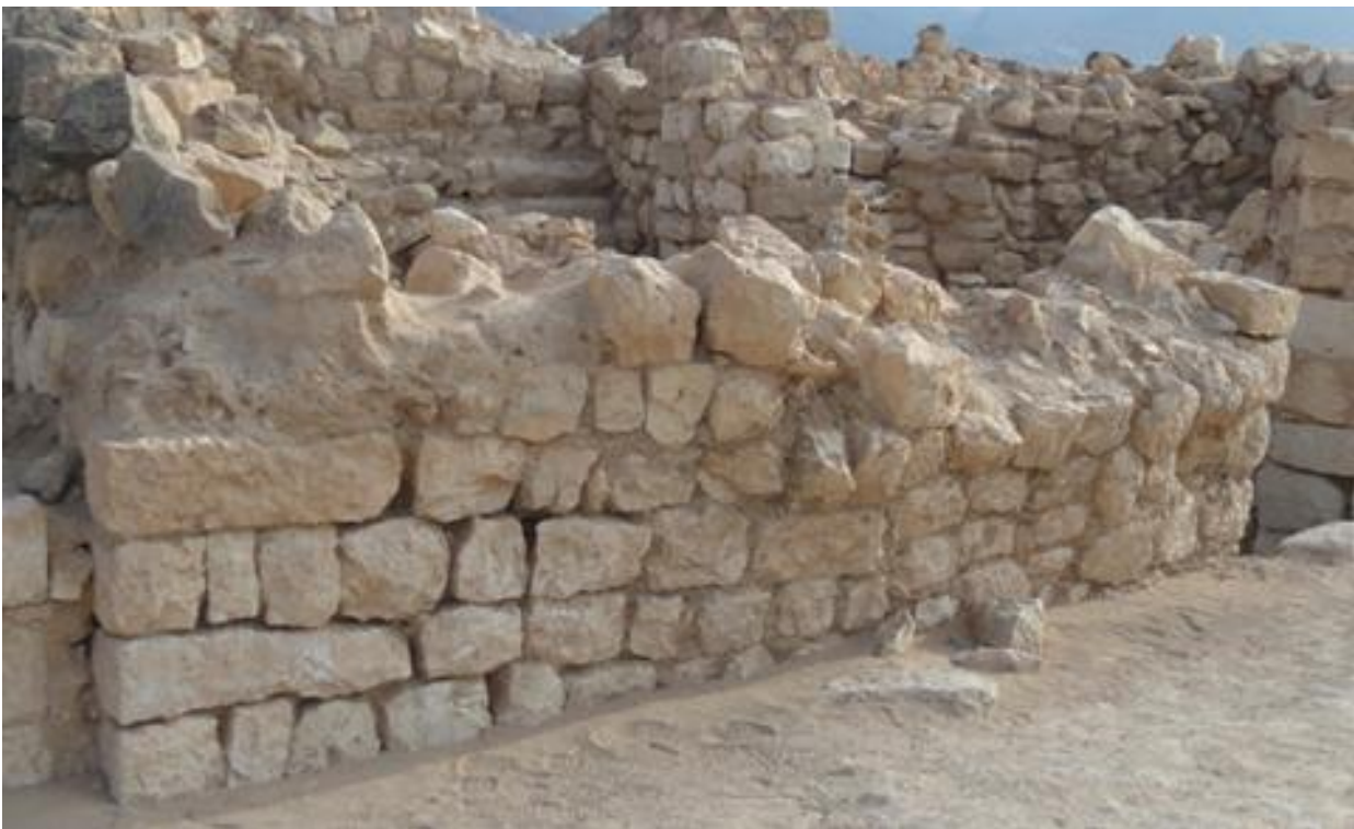
M635, south front wall, before the restoration.
