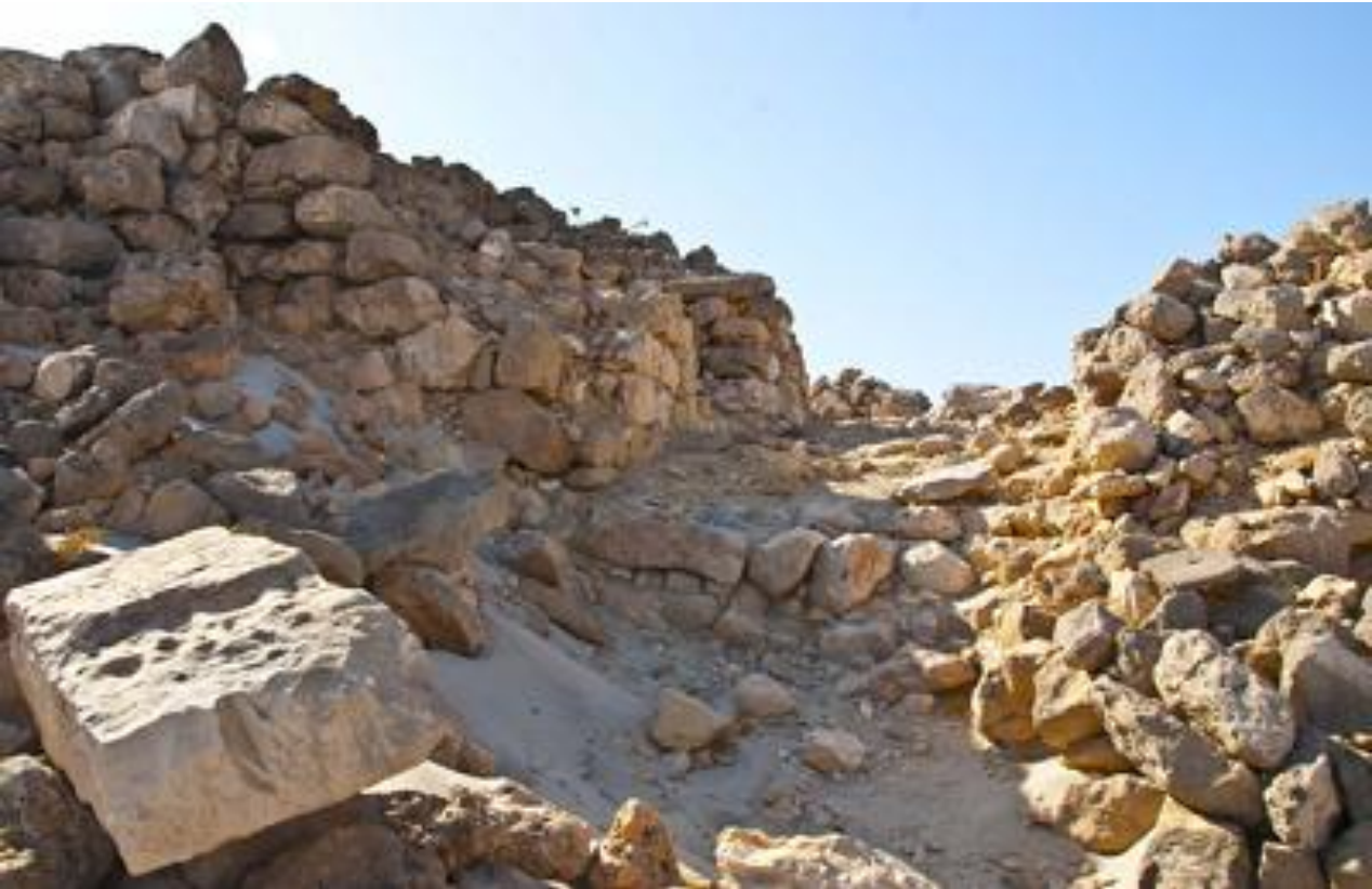
Principal door north side before restoration
