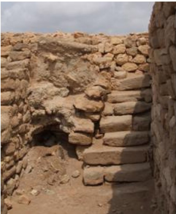
M63, south front wall, before the restoration.
