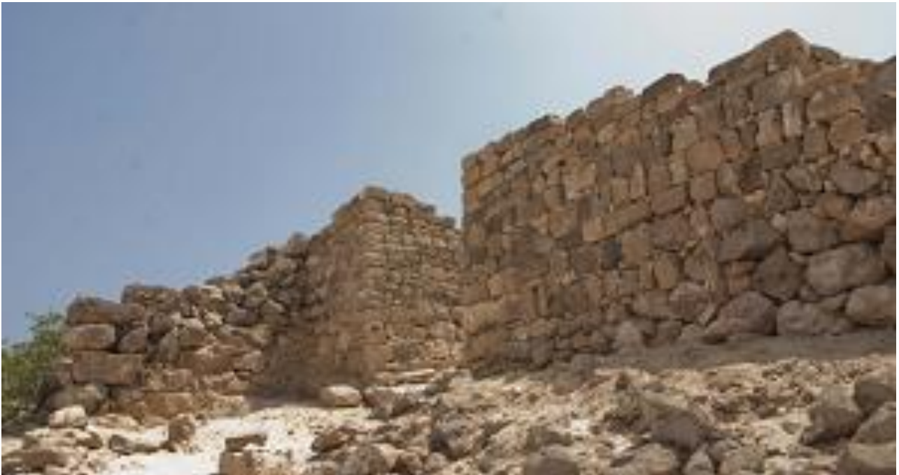
View on the up street after restoration
