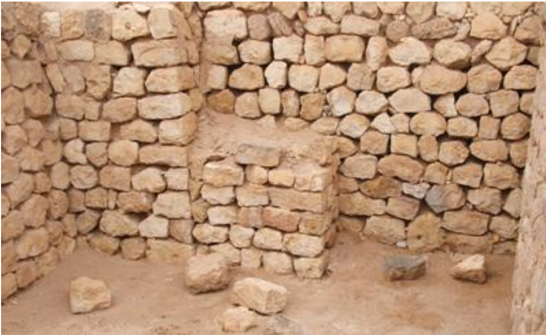
M69, south front wall, before the restoration.
