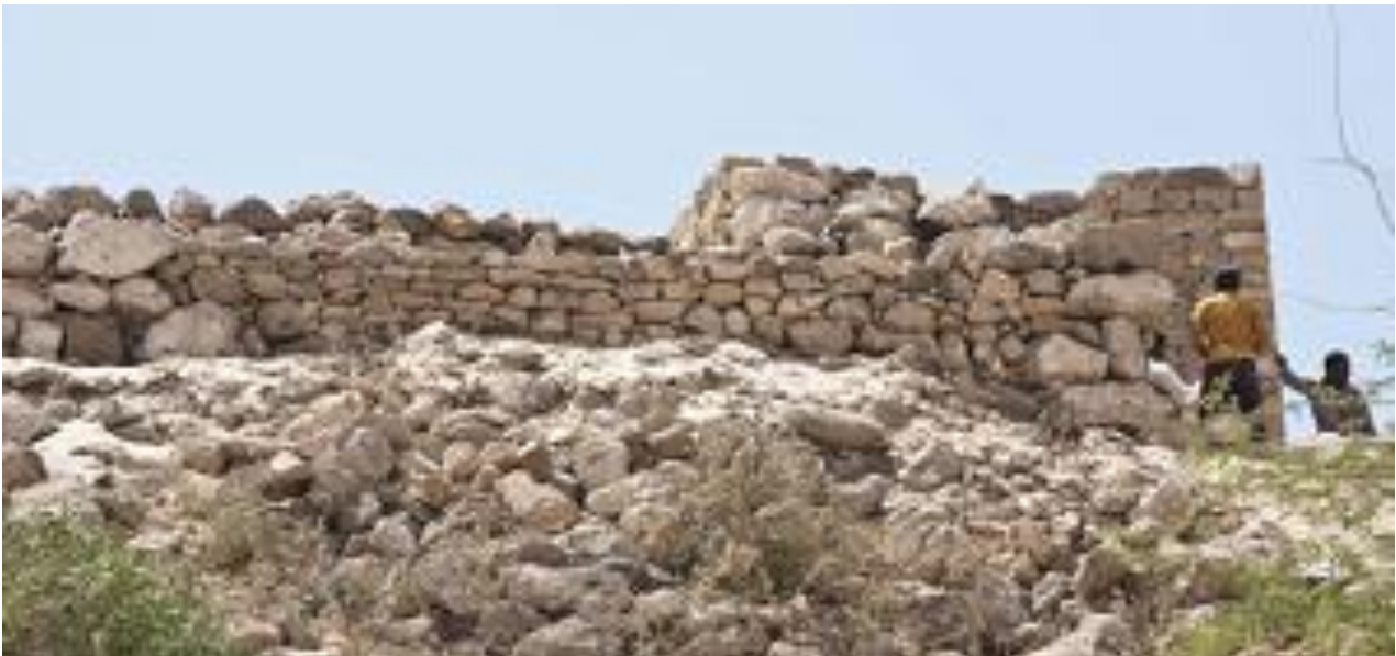
View north side after restoration
