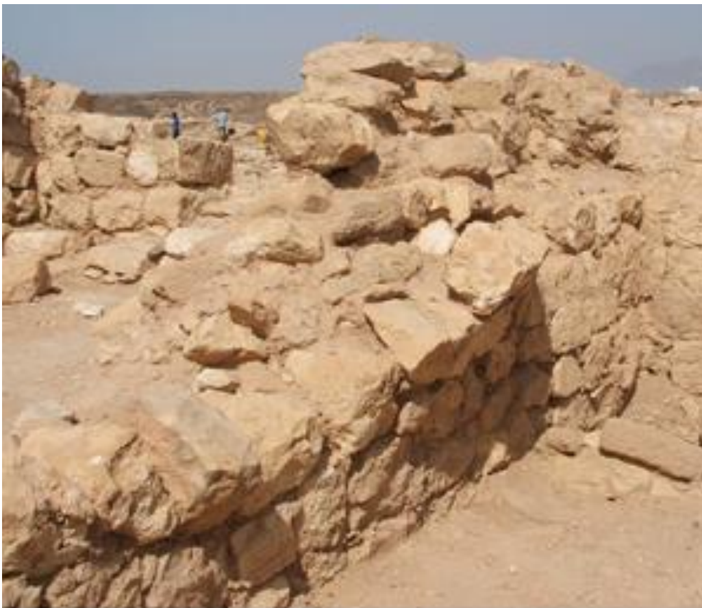
M529, north front wall, before the restoration
