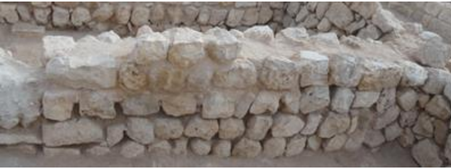
M569, north front wall, after the restoration.
