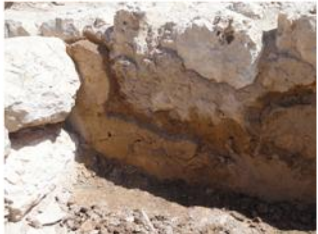
Setting of new plaster
