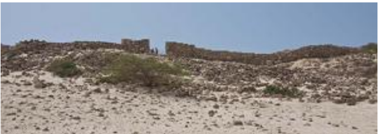
View on the principal street, north side east wall, east tower, west tower and west wall
