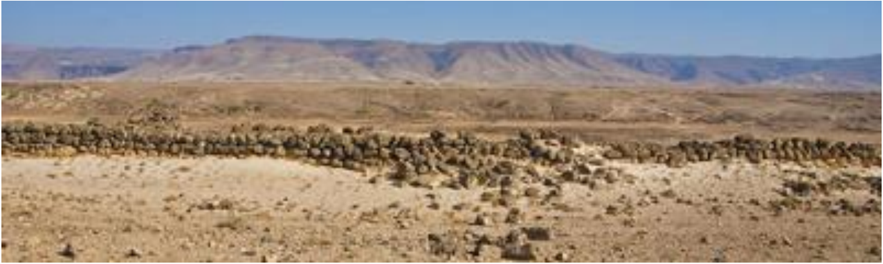
West wall in bad condition
