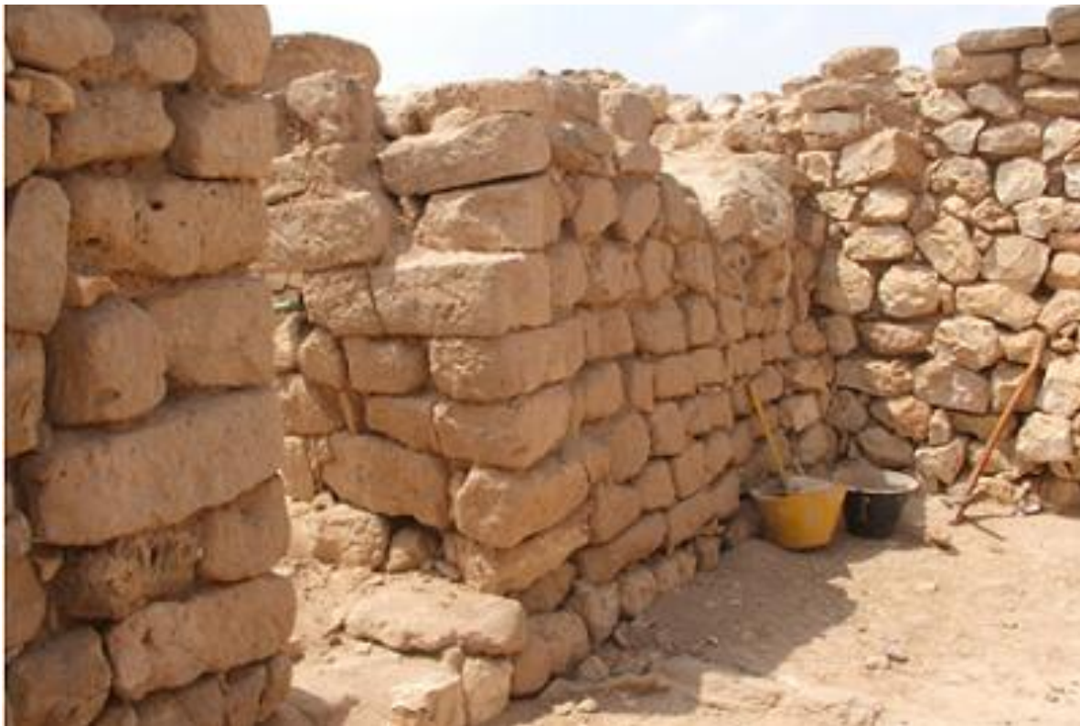
M70, south front wall, before the restoration.
