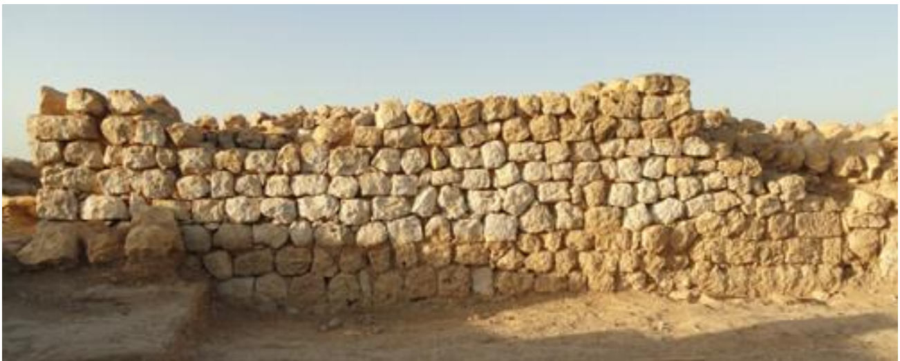
M485, south front wall, before the restoration.
