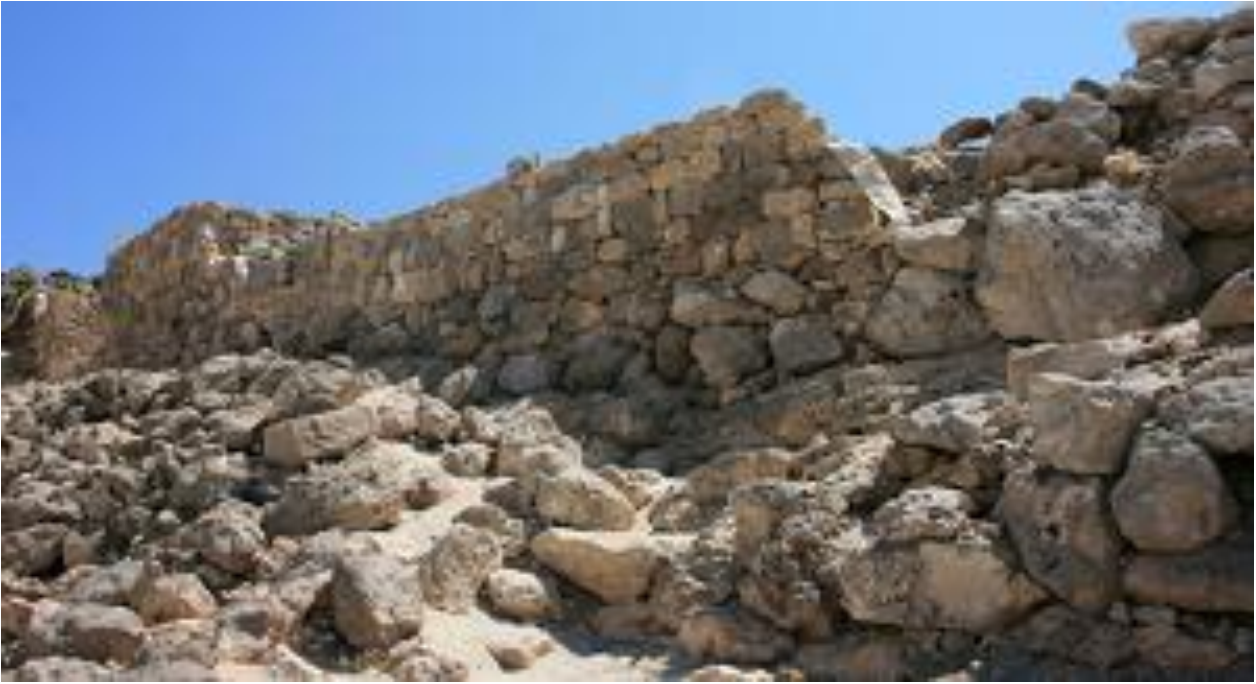
Northern face during restoration
