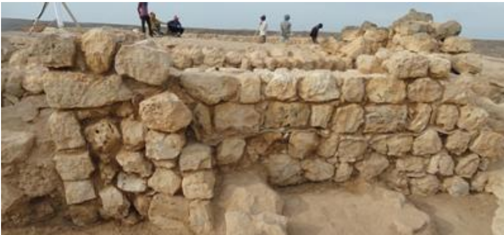
M567, south front wall, after the restoration.
