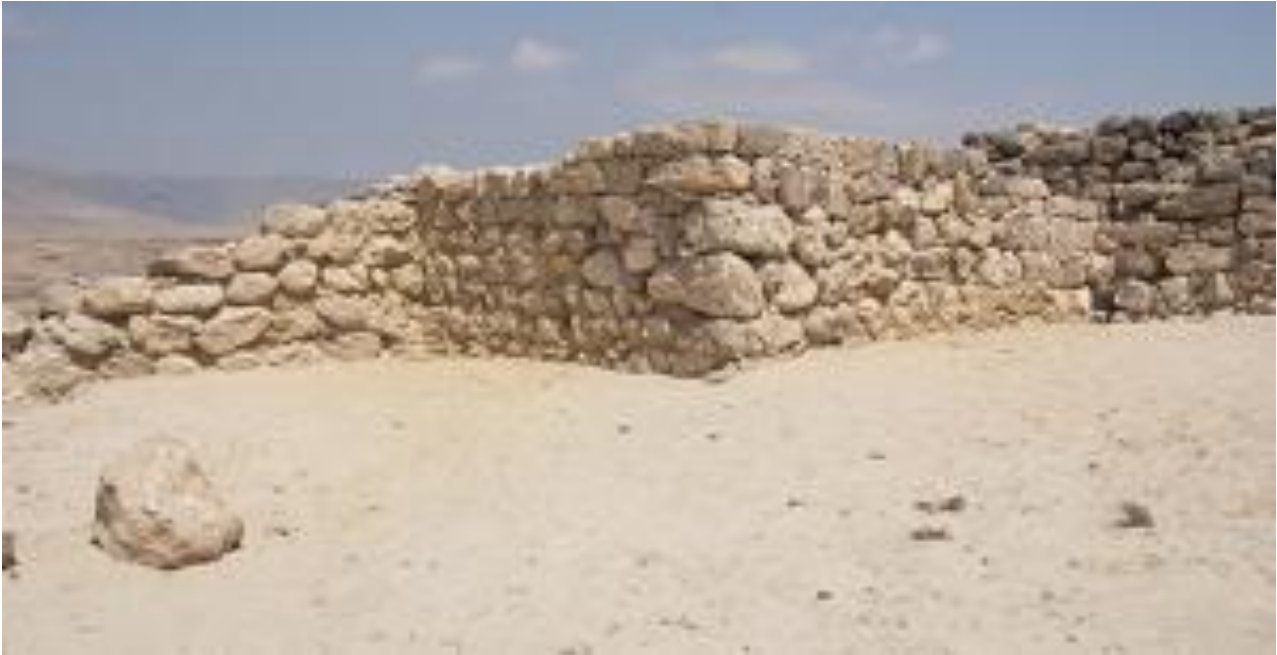
South - East side after restoration
