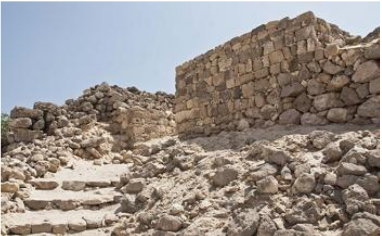
View on the up street before restoration
