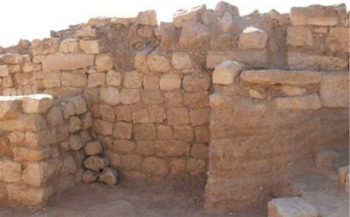
M521, west front wall, before the restoration
