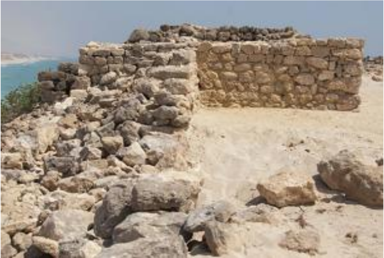
East side after restoration
