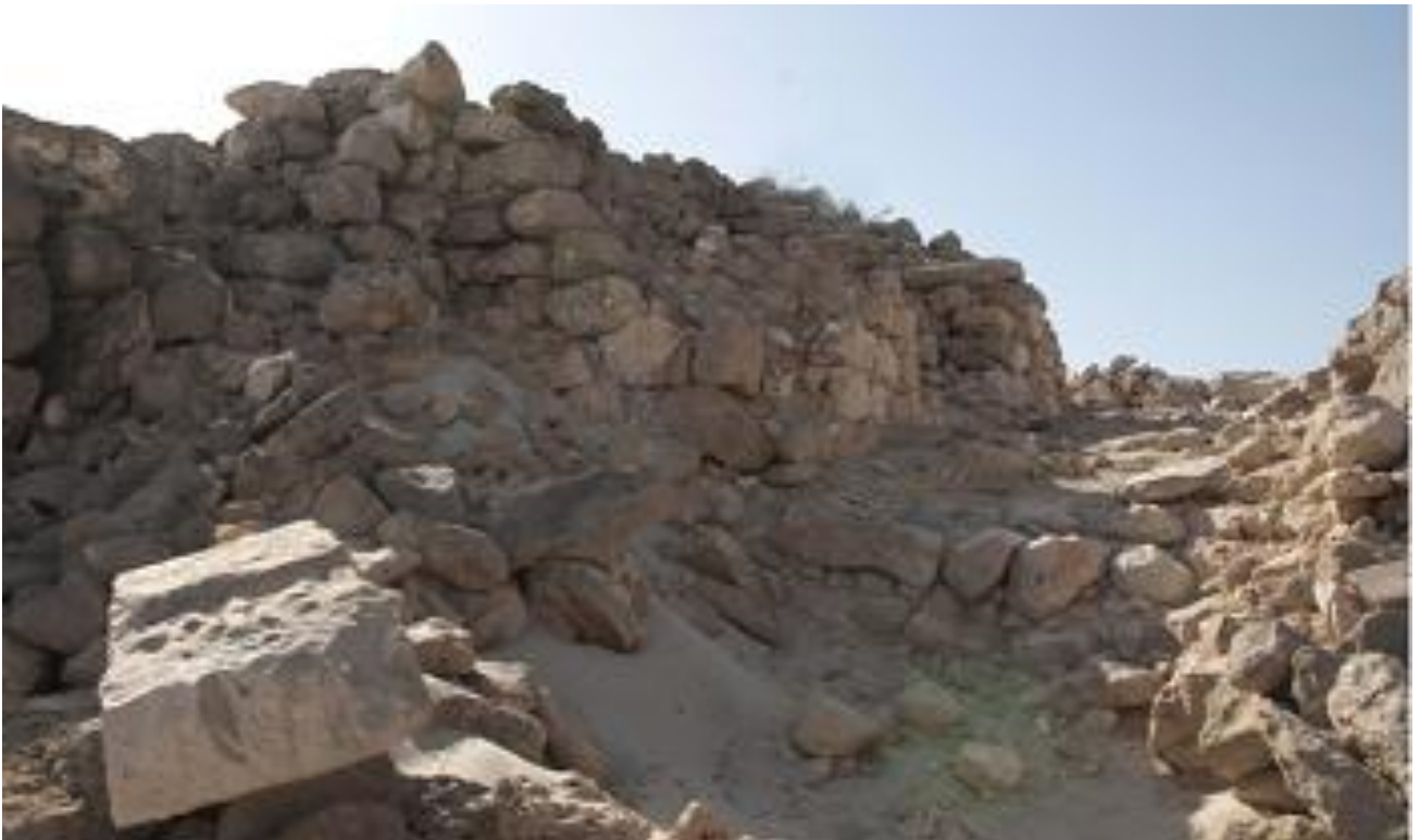
View north-west side before restoration
