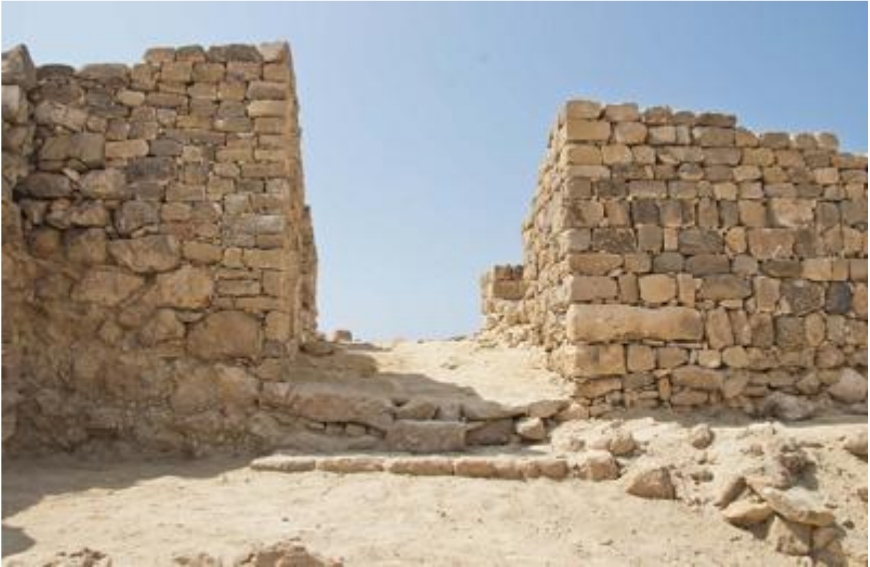
Principal door north side after restoration
