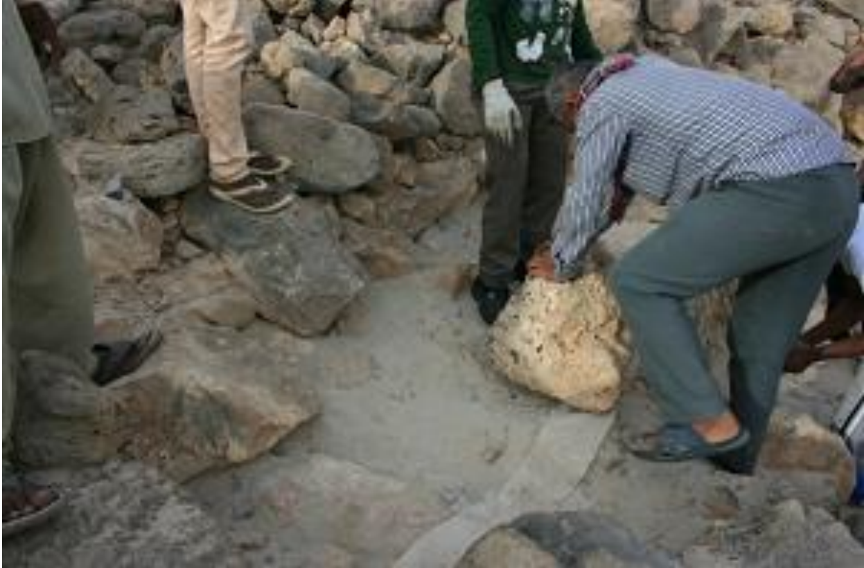
Consolidation of basement
