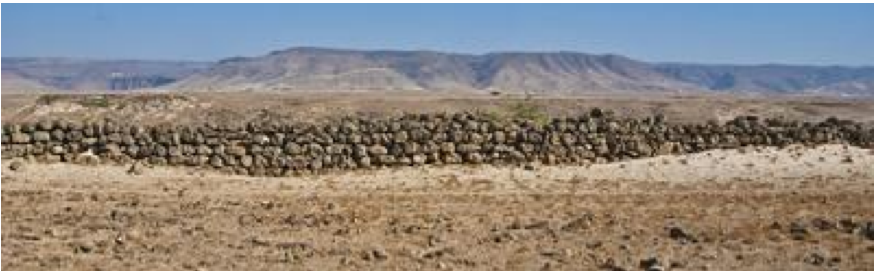
West wall in good condition
