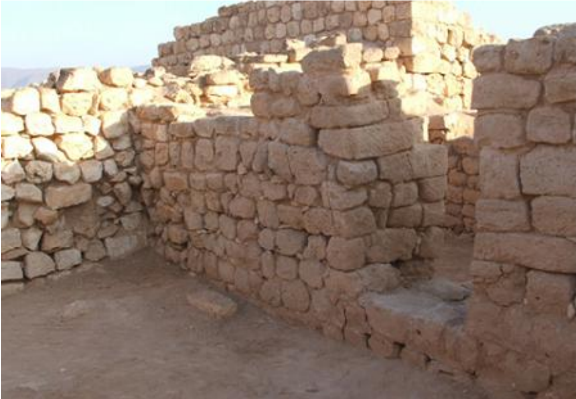
M70, south front wall, after the restoration.
