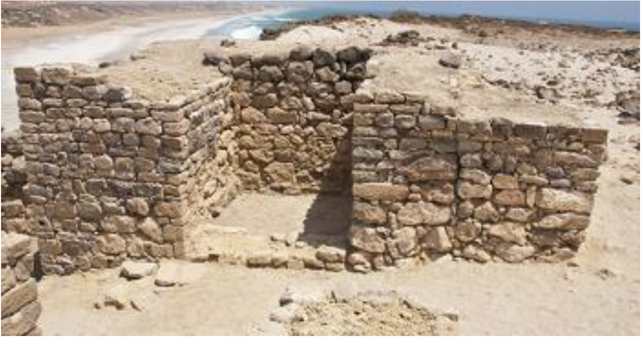
View east side after restoration
