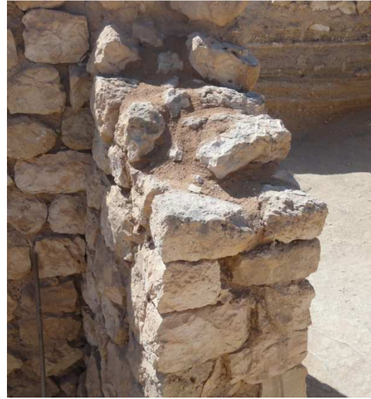
M290, before and after the restoration.
