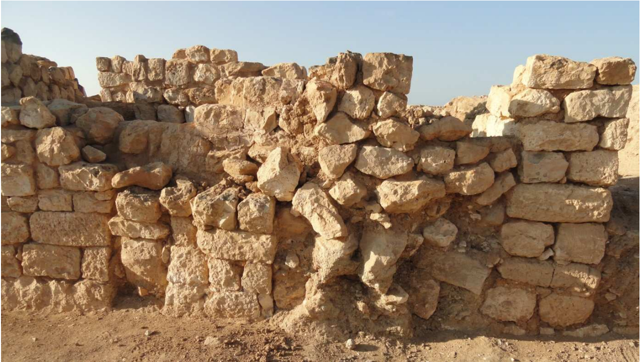
M485, North front wall, before the restoration.
