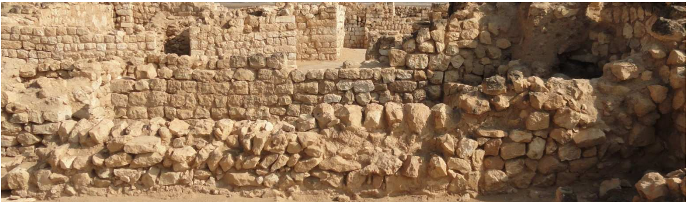
M582, South front wall, before the restoration.
