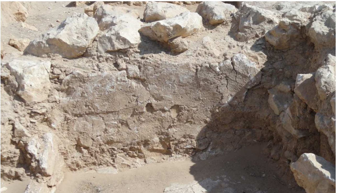
South wall, façade. before the restoration
