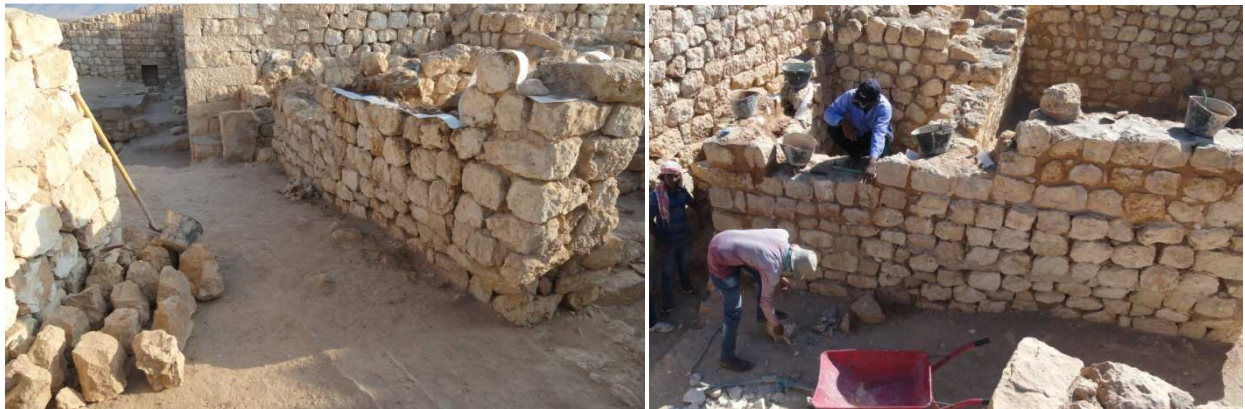
M290-274, West front wall, during the restoration work.
