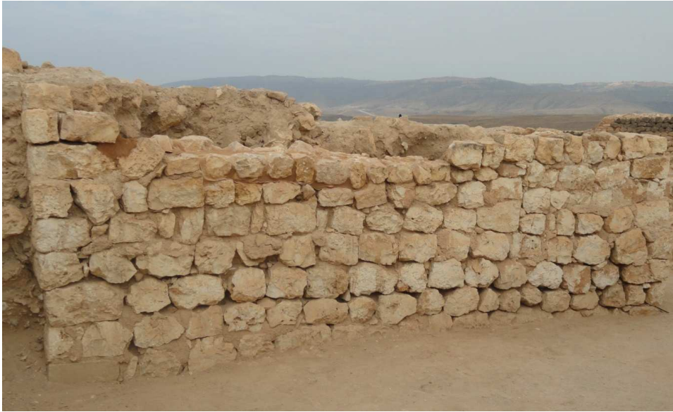
M464, East front wall, after the restoration.
