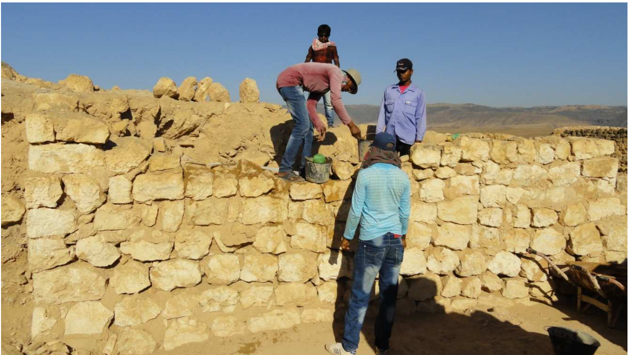
M464, East front wall, during the work.
