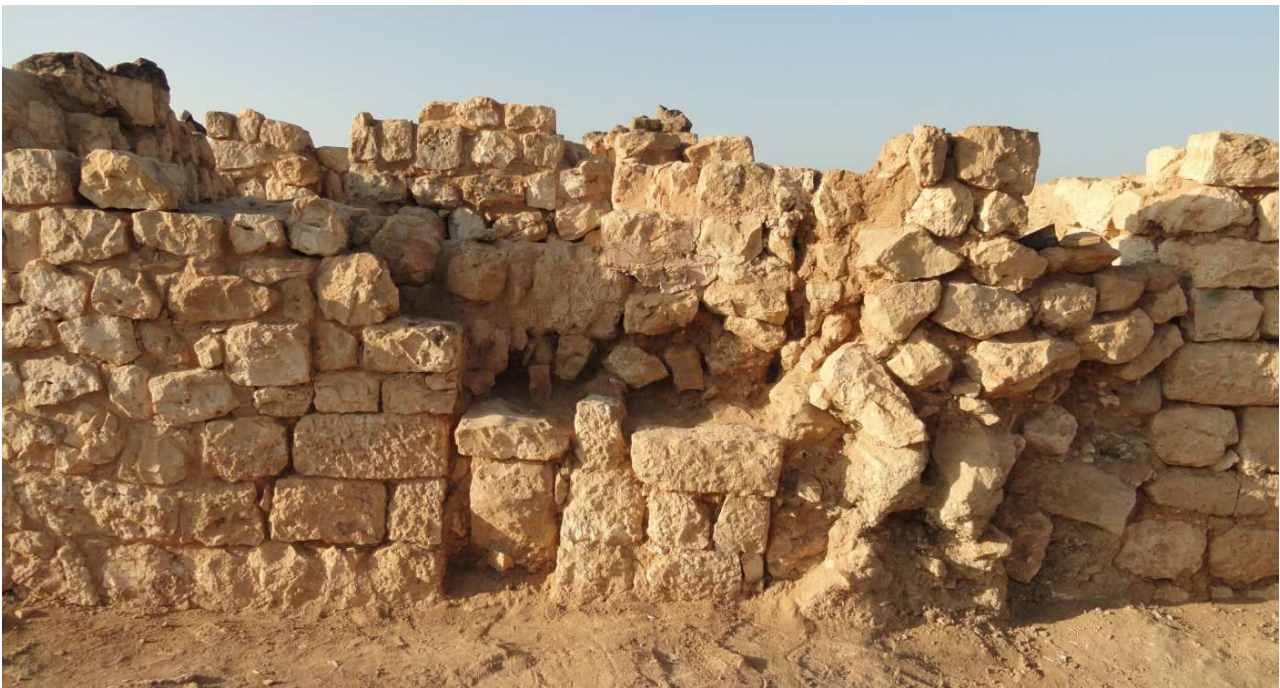
M485, North front wall, during the cleaning work.
