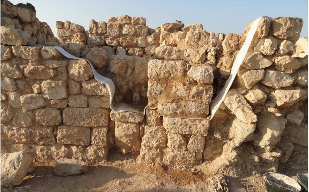
M485, North front wall, during the restoration work.
