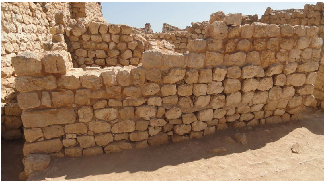
M290-274, West front wall, after the restoration.
