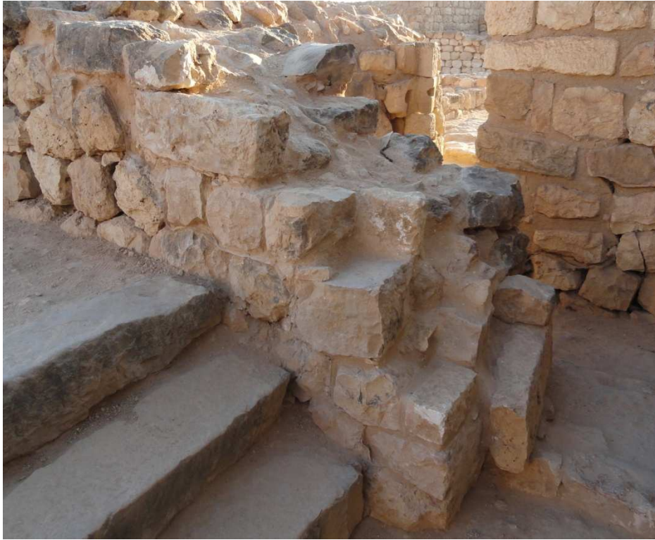
M16, West front wall, after the restoration.
