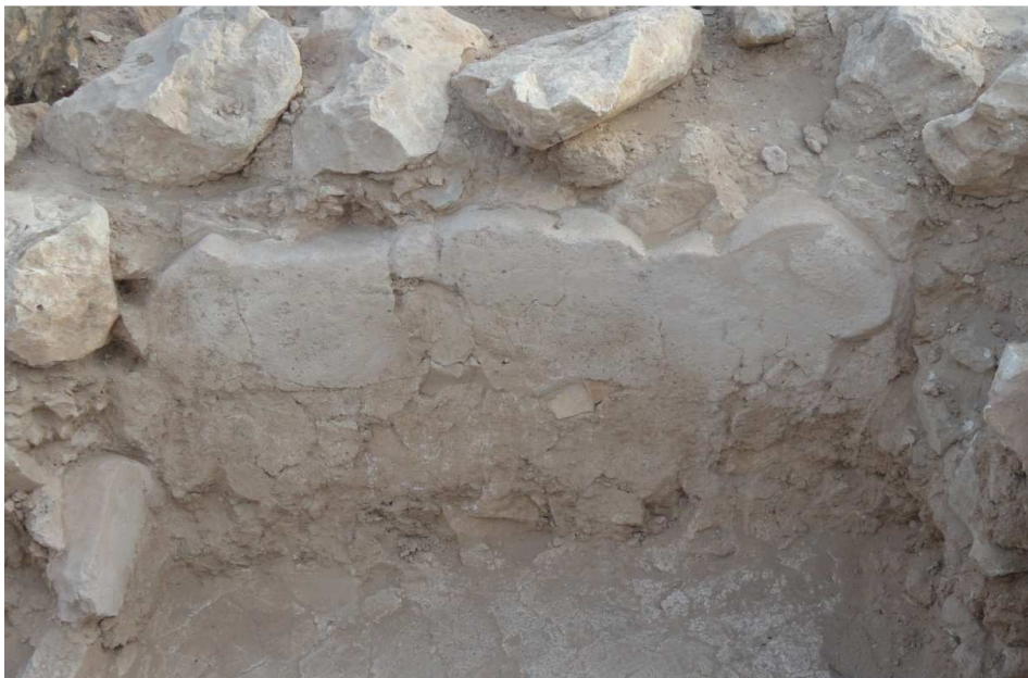
South wall, façade. after the restoration
