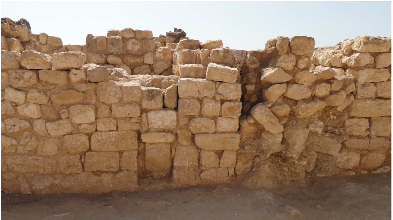
M485, North front wall, after the restoration.
