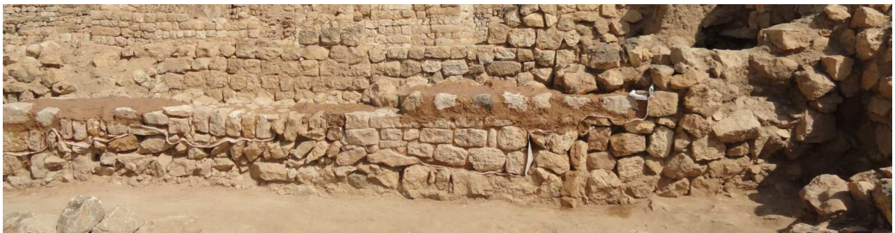
M582, South front wall, during the restoration work.
