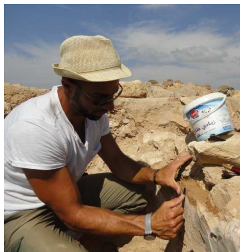
Setting of new plaster
