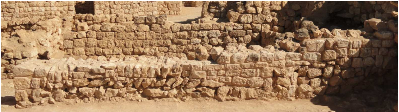
M582, South front wall, after the restoration.
