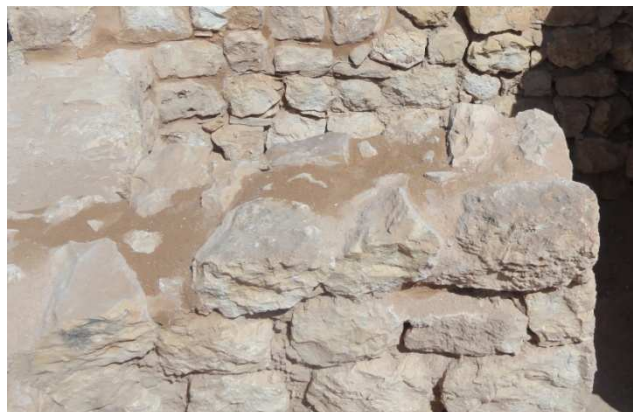
M400, before and after the restoration.
