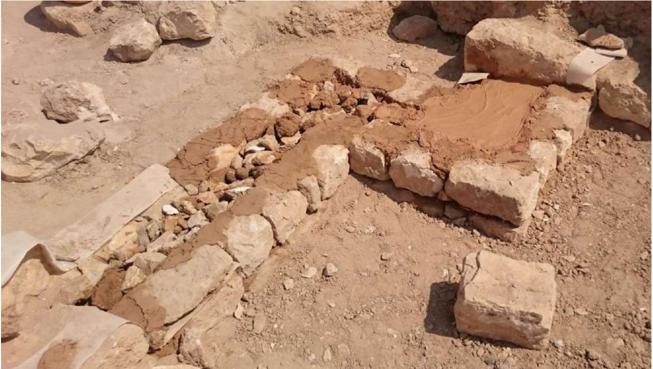
Fig. 5 – Realization of a new masonry wall, with the two outer faces in rough stone blocks and with the core filled with small stones and mortar. Building BB4, wall M646.
