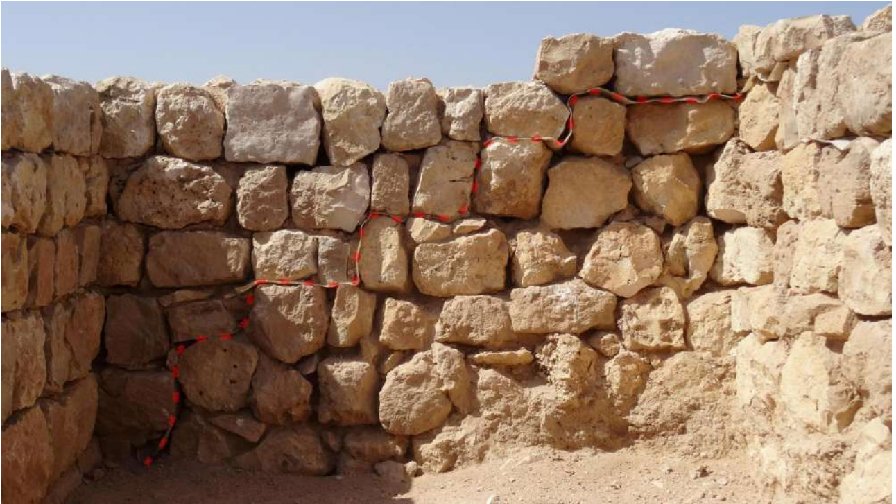
Fig. 3 – New (on the left) and old (on the right) masonry texture. Building BA12, wall M185.
