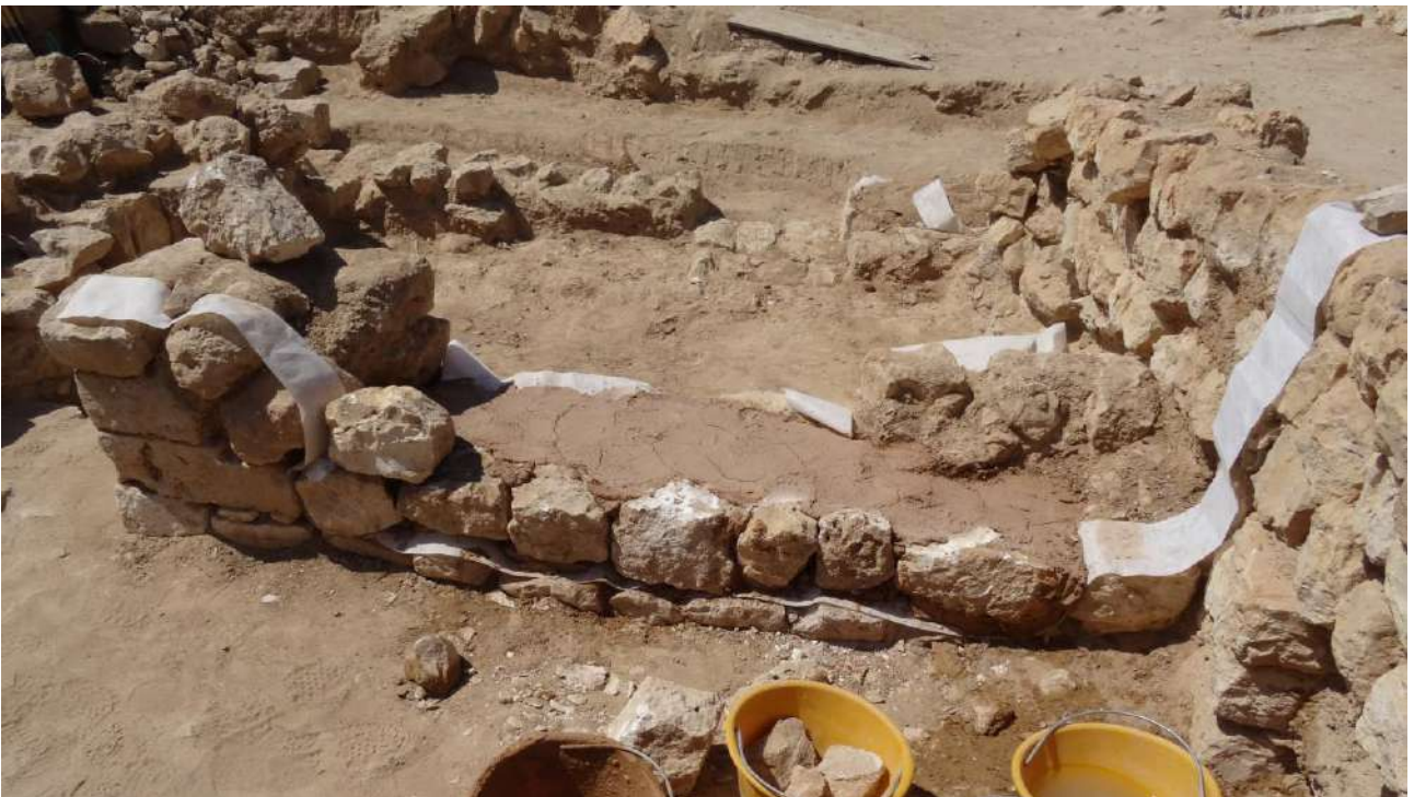
Fig. 4 – Geotextile layer placed between the original masonry and the reconstructed wall. Building BB4, wall M645.
