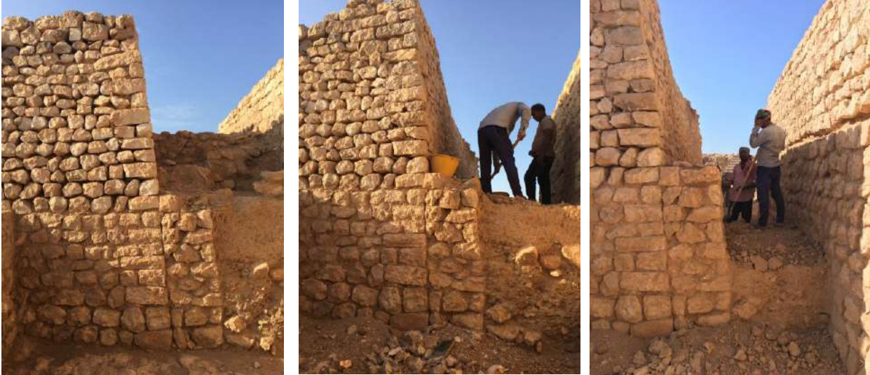
Dismantling and removal of walls.
