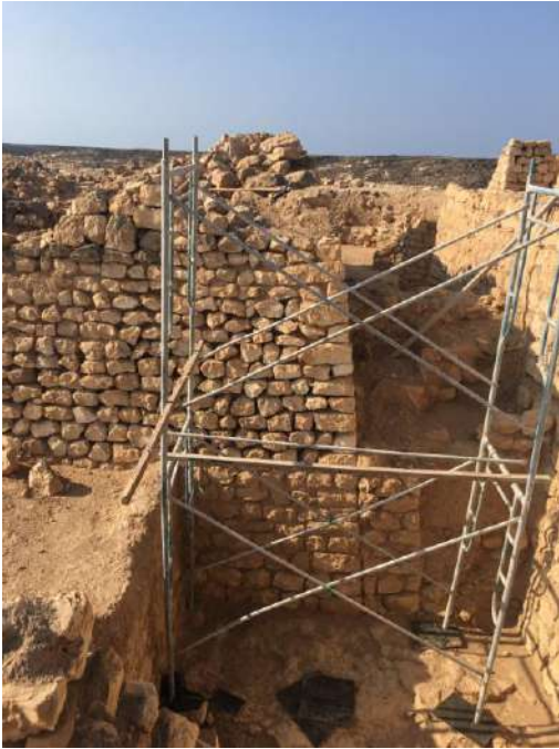
Scaffolding assembly and cleaning with partial removal of the stones.
