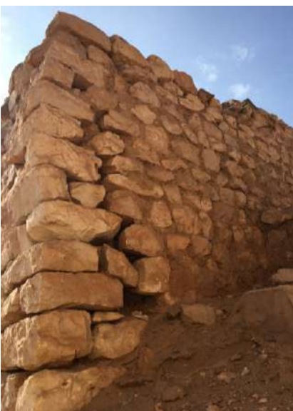
Corner wall, before the restoration. The fracture along the masonry
