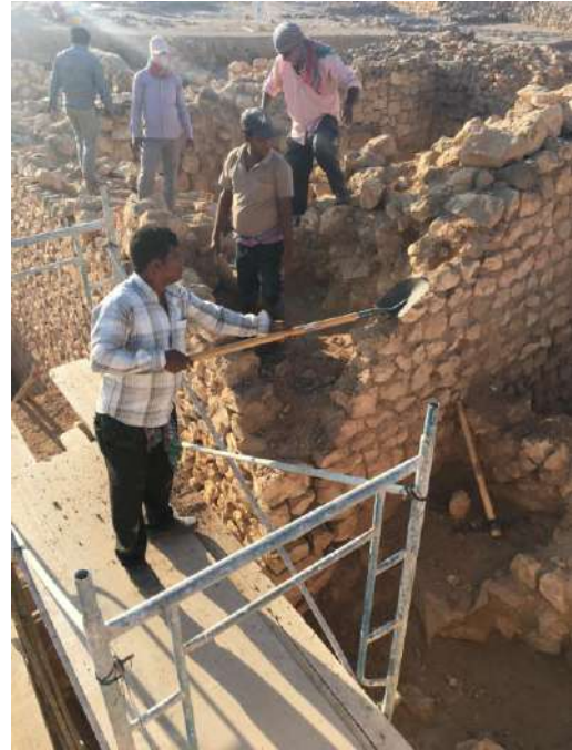
Scaffolding assembly and cleaning with partial removal of the stones.
