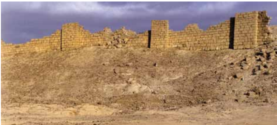
Fig. 5 - Baraqish (Main), city walls
